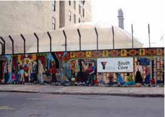
Parcel R-1 was the site of the former Chinatown YMCA.
