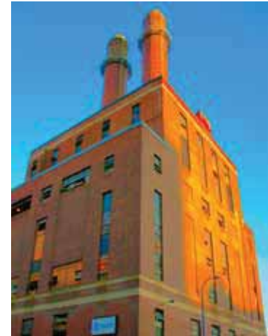
Trigen Energy Plant on Kneeland Street.
