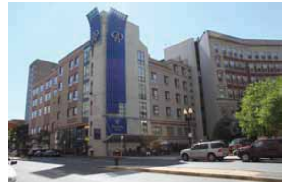
The former Don Bosco High School was redeveloped as the Doubletree Hotel and Chinatown Wang/YMCA in 2000.
