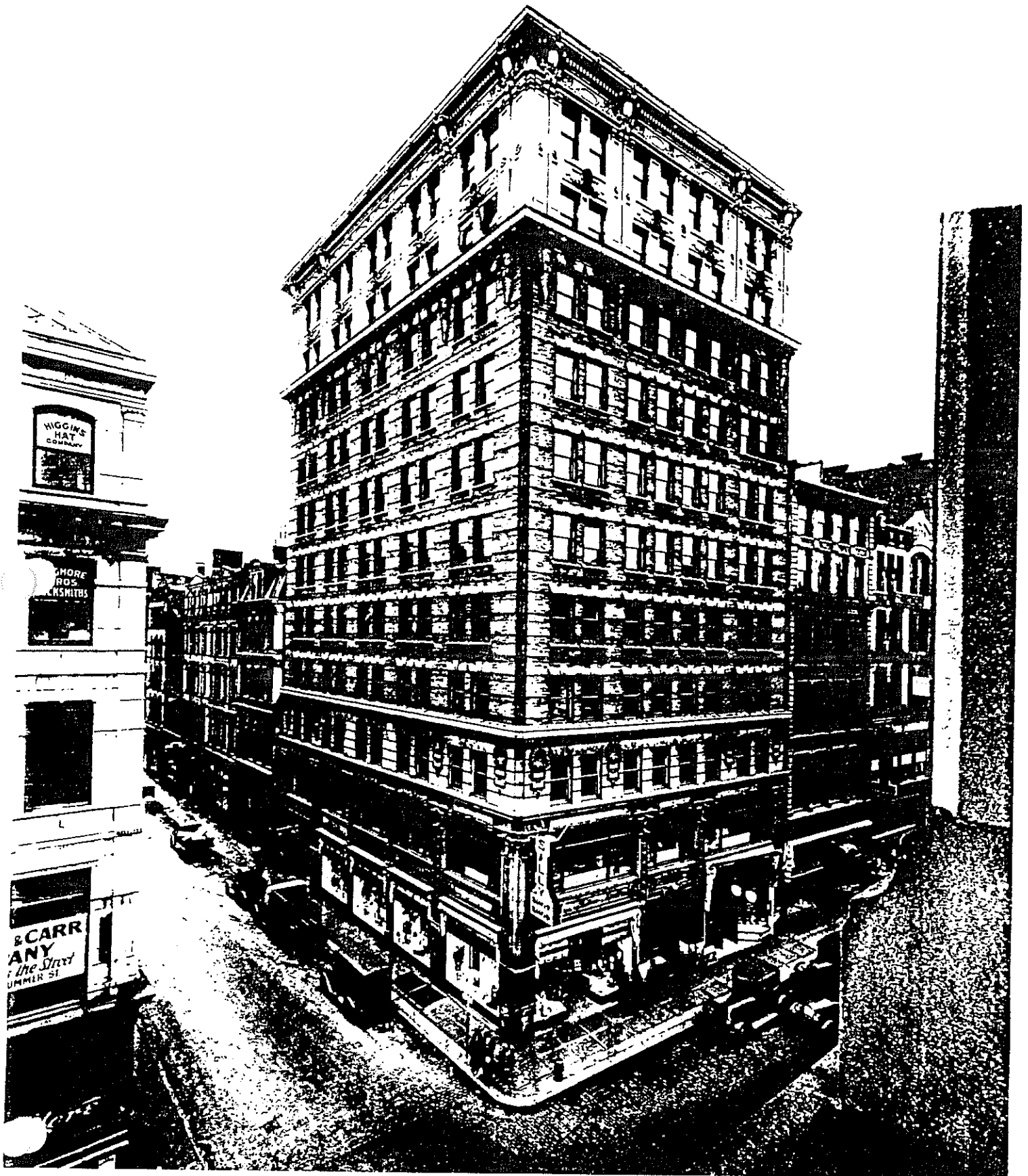
MERCHANTS BUILDING 75-81 Summer Street aka 3 Kingston Street ca. 1928 Bostonian #4220
