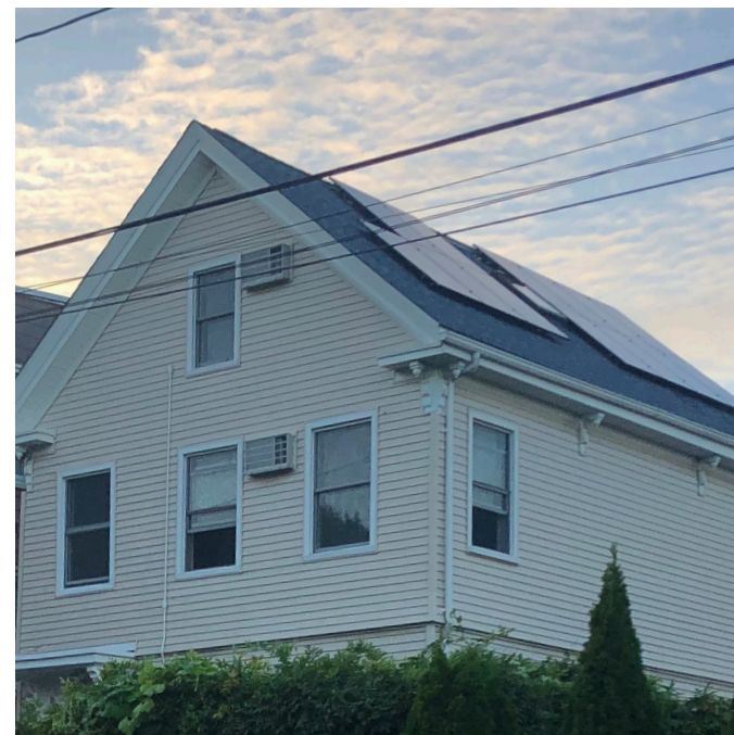
Vents and other mechanical elements should be located away from the primary facade of the building. The exception is photovoltaic panels, which are encouraged both on flat and pitched roofs and on the ground level of the site.
