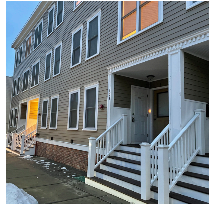
Entrances should be clearly visible. In East Boston, many entrances are recessed, and so proper lighting and visibility from the street should be prioritized for the safety and security of occupants.
