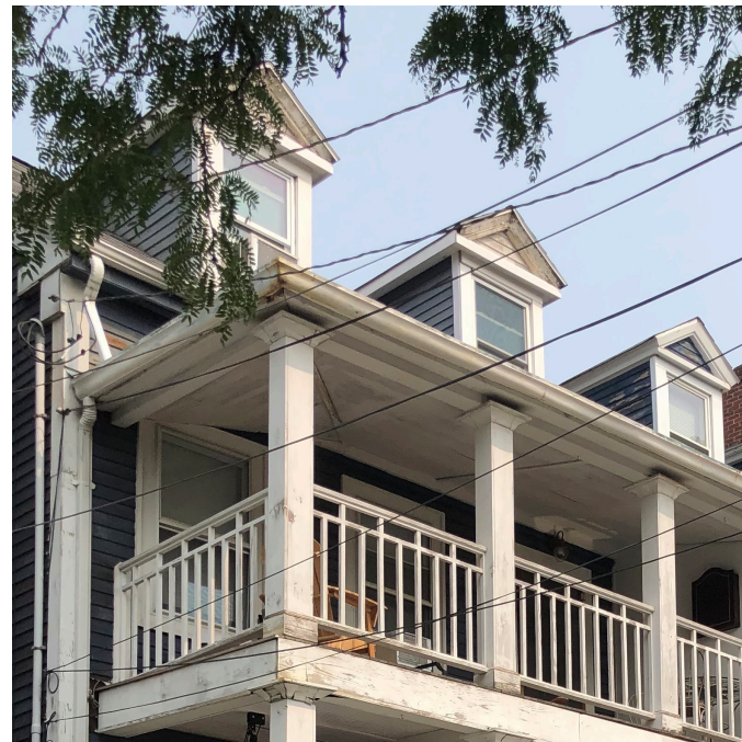
Massing variations such as porches can create interesting contrasts and/or connections to the main building volume. Secondary elements such as columns, railings, and edging should be scaled appropriately and should use materials that complement the building facade.
