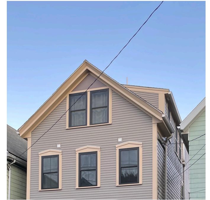
The treatment of additions depends on the context. Small additions may be treated in a similar manner to the existing building, such as the shed dormer above.
