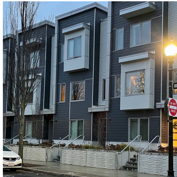
Buildings with elevated first floors may use facade articulation, planting, or other strategies to create an active edge.
