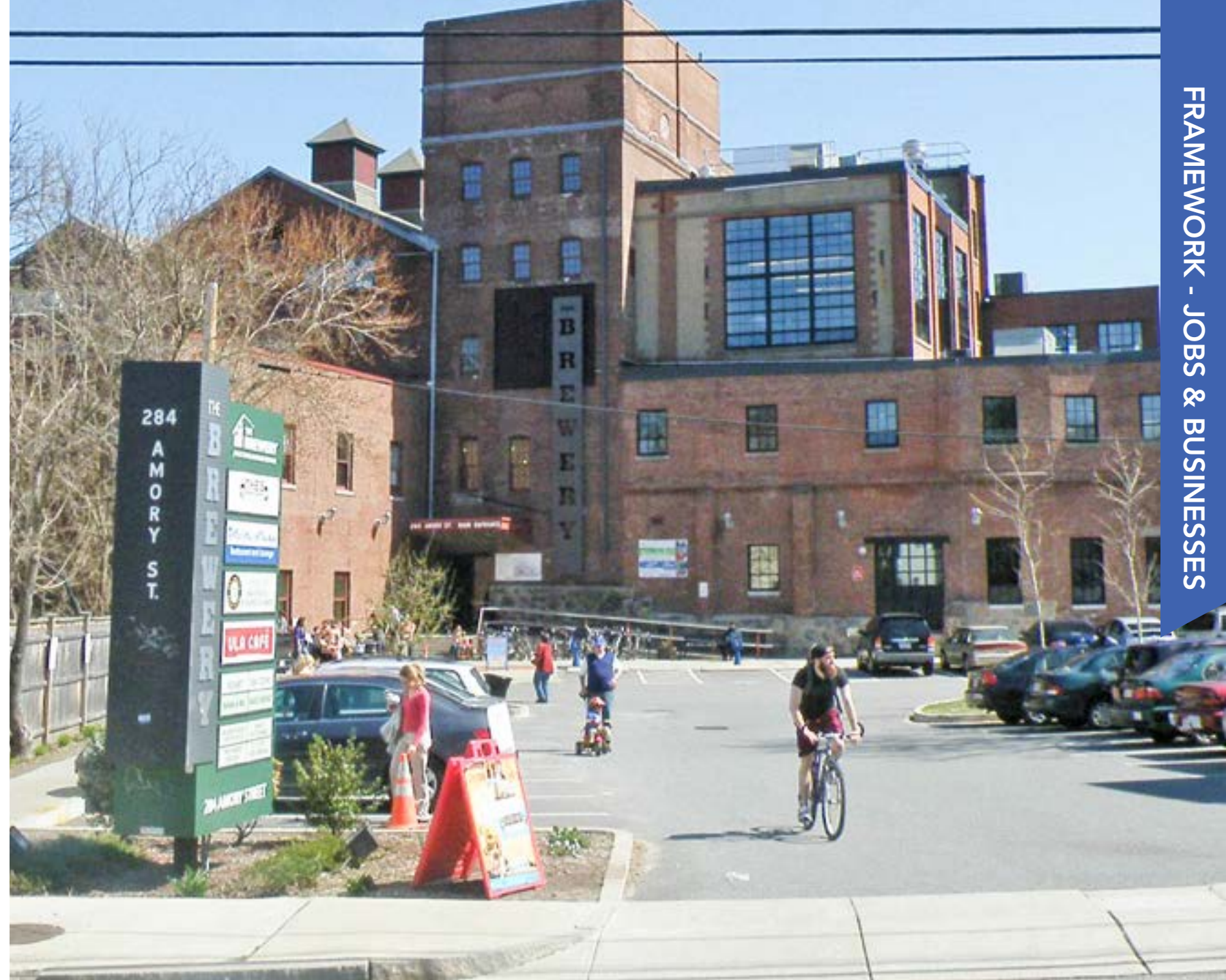
Figure 25. The Brewery Complex, renovated by the Jamaica Plain Neighborhood Development Corporation, contains approximately 40 businesses and services within 4 different buildings.
