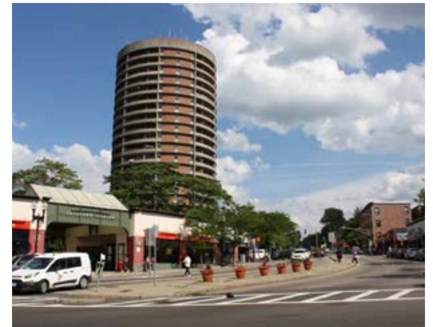
Figure 18. Walnut Park Apartments, a 168-unit public housing development for seniors and people with disabilities ("Roundhouse")
