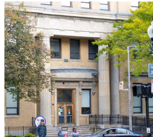
Roslindale Community Center
