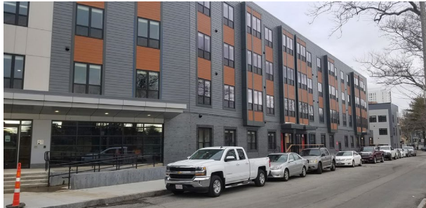
Whittier St Housing I 3 to 4-story, 45ft height 92 units
