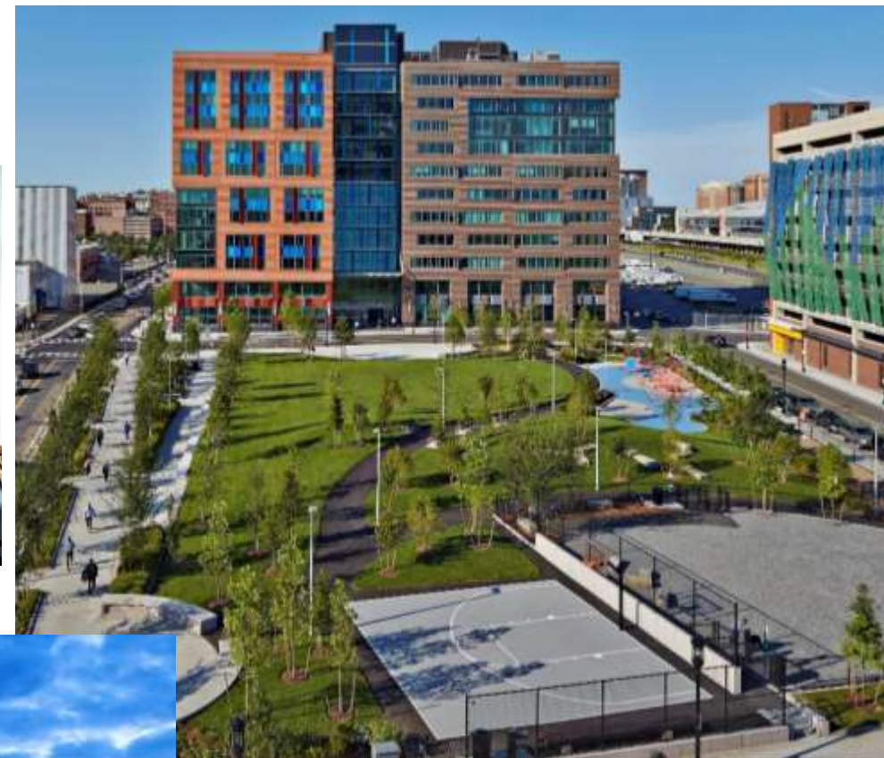
A Street Park. State Street Headquarters. South Boston.
