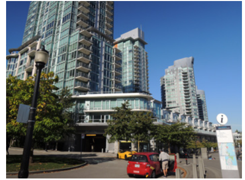
Figure 165. A series of towers are linked by a common podium that is active in use along the main pedestrian thoroughfare, Vancouver, BC.
