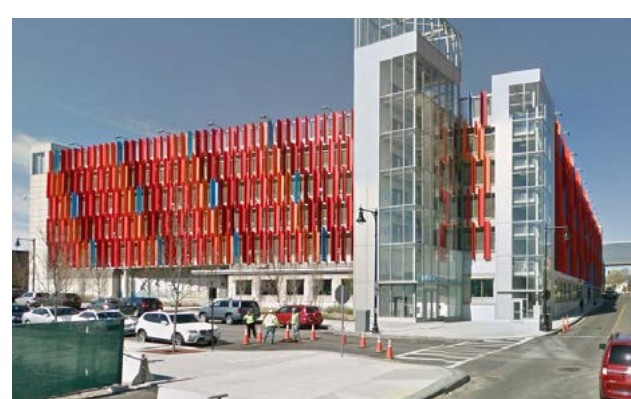
Left: Examples of how parking garages should either be screened or wrapped with active uses Right: Parking Garage Design Guideline Diagram
