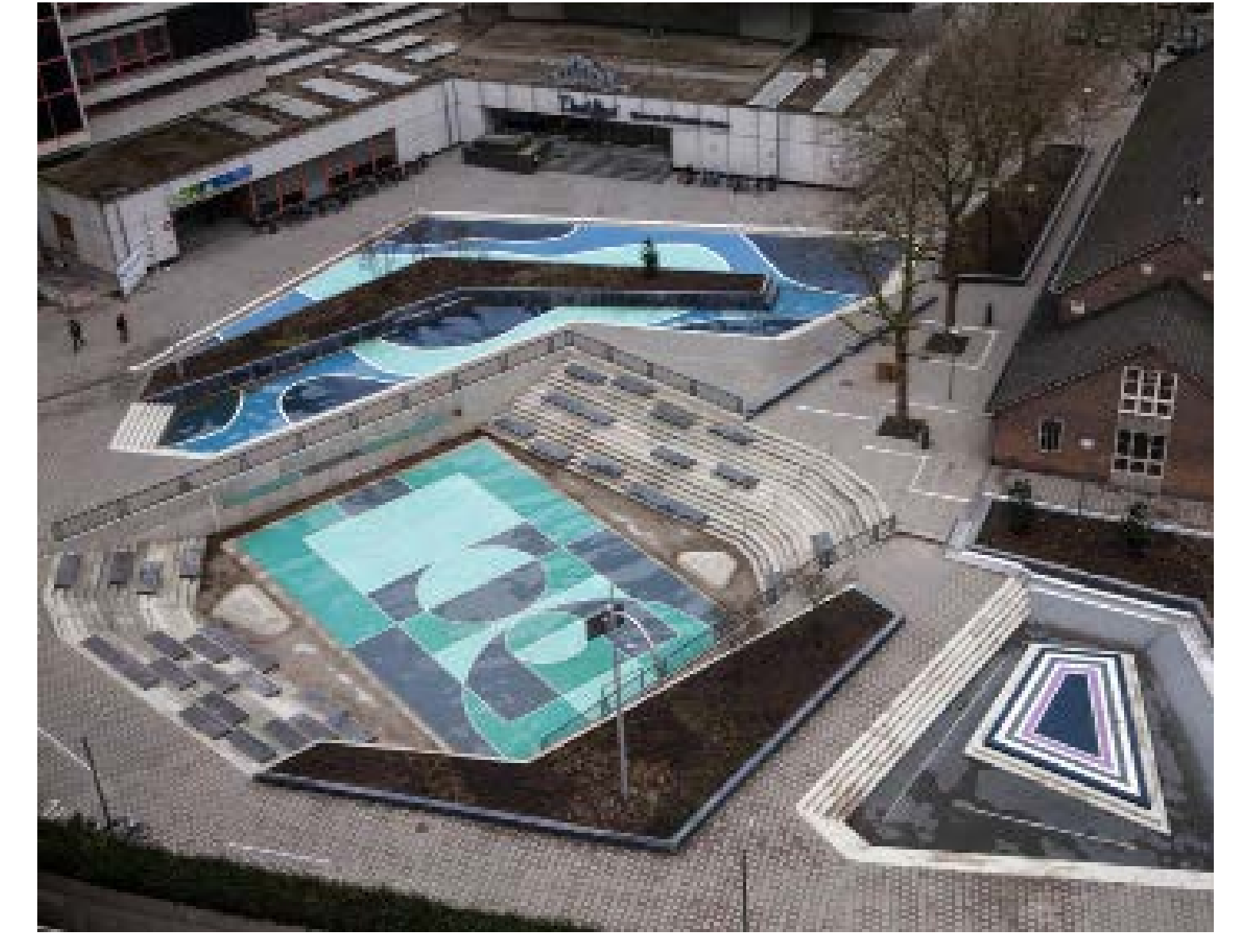
A sub-level park and flood resiliency tool that fills up with runoff during heavy rains, Rotterdam
