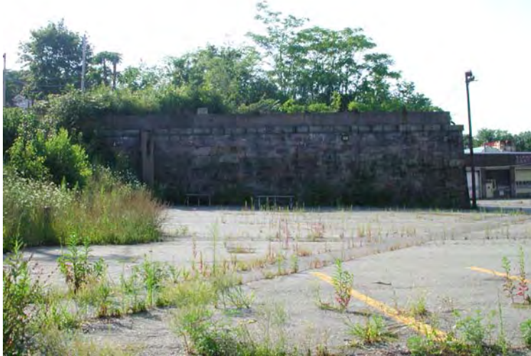
Washington St. at Guild / Retaining Wall
