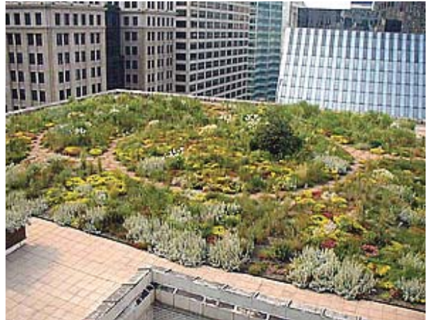
Green roofs add to the character and mitigate the effect of hard dark surfaces on the urban environment.
