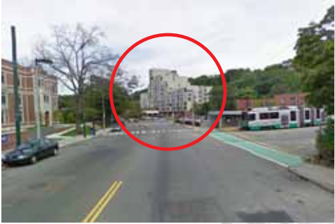
D. South Huntington Ave. View - Back of the Hill Apartment
