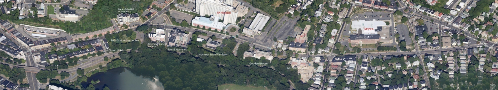
S. HUNTINGTON AVE. CORRIDOR AERIAL VIEW LOOKING EAST
