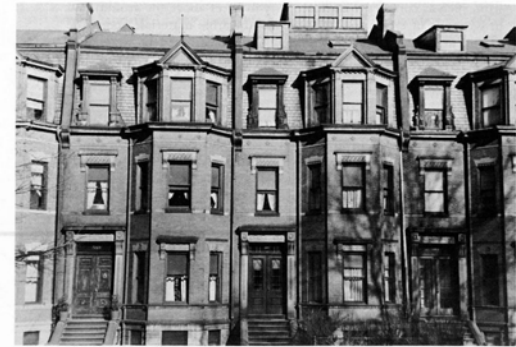
160 Facade of 385-389 Marlborough Street, 1880, by O. F. Smith. When compared with similar sized houses of 1863, fig. 29, these facades illustrate how bay windows and other appendages destroy the continuity of later rows of houses. The gutter stones and fire walls were required by fire laws.
