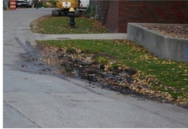
area of subsidence; pavement caving in; soils likely do not have structural capacity to support use;
