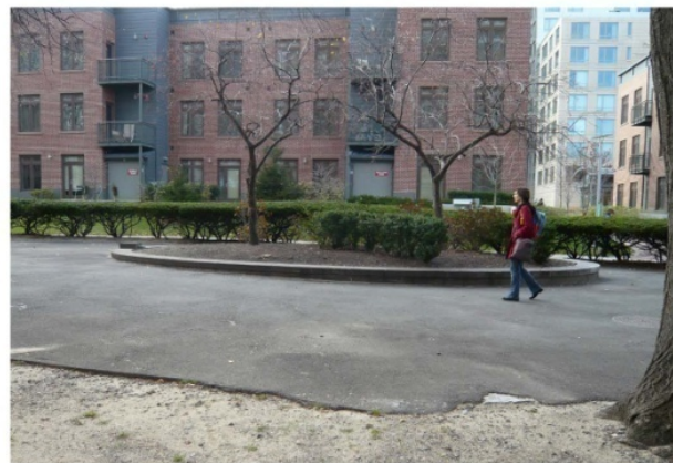
major areas replaced with asphalt paving
