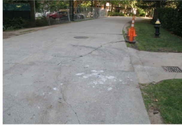
area of subsidence; pavement caving in; soils likely do not have structural capacity to support use;
