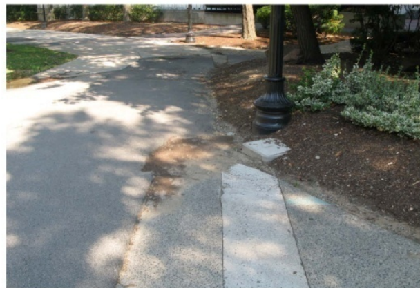
patches for utilities added to pathway
