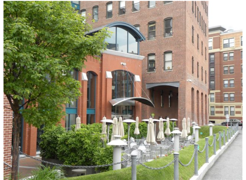
560 Harrison Ave after
