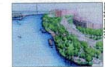
The new Nashua Street Park, currently under construction, will extend the Charles River Basin park system.
