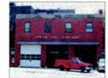
Public safety facilities, such as fire and police stations, must be an integral part of community planning.
