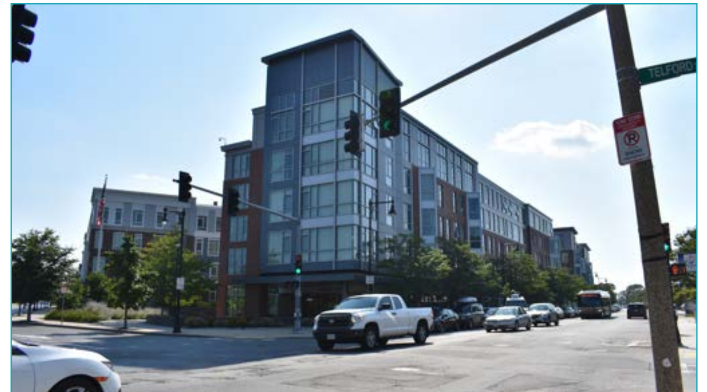
Charles View Apartments
