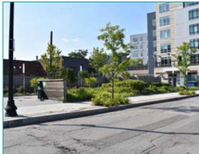
Open space created as part of the 180 Telford Street residential development
