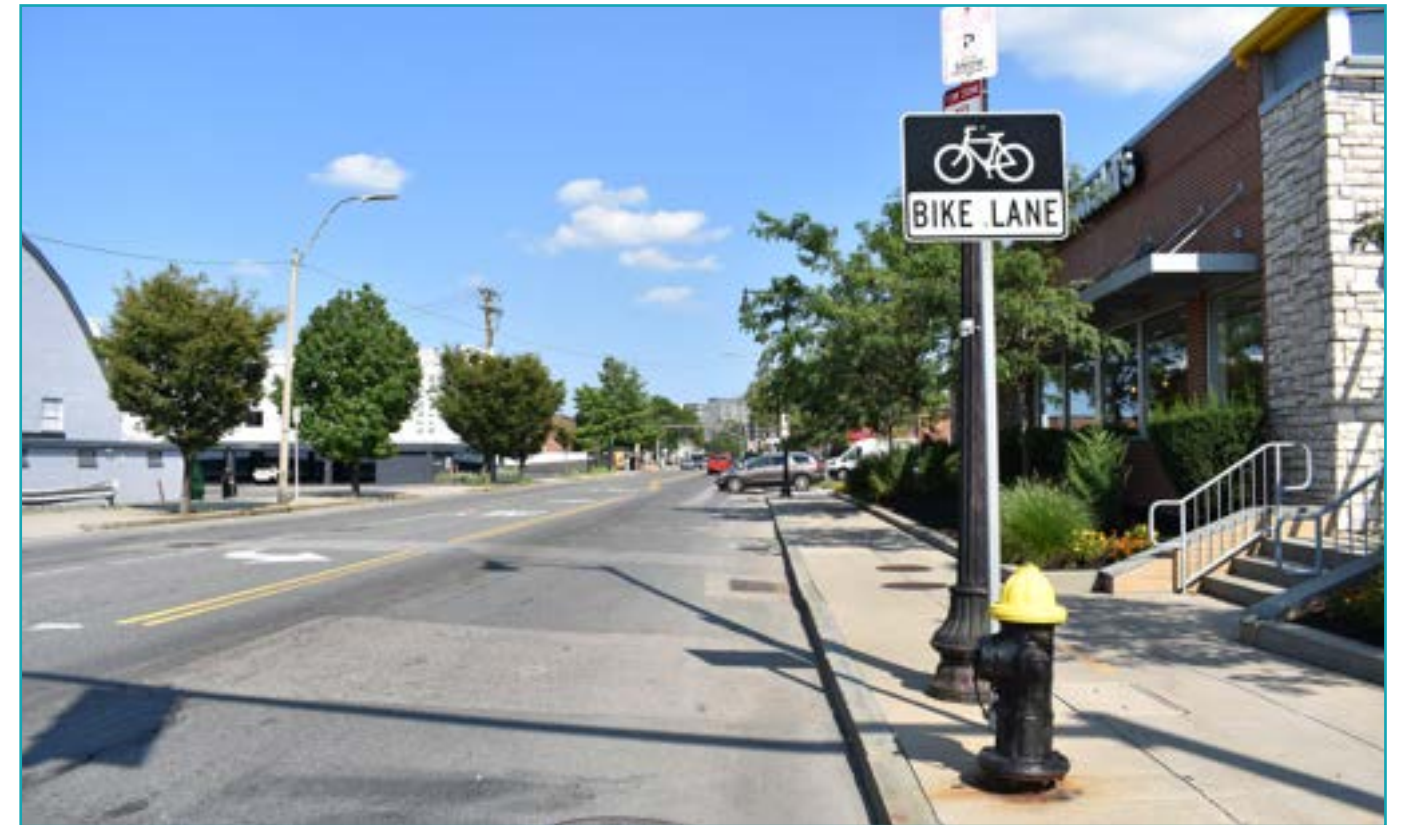
Bike Infrastructure on Western Avenue today. Bike lanes are marked with signage, but space is not marked or designated on the roadway itself.
