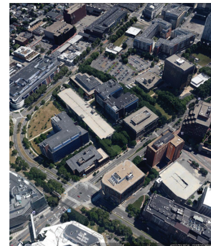
Hidden from sight and sound, the Biogen energy plant is nested beneath a research building in the Kendall Square area. Photo credit: Google Earth
