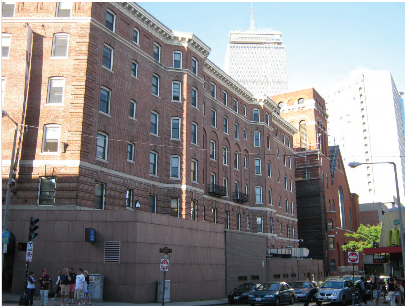
Figure 4-10 150 Massachusetts Avenue Existing Conditions
