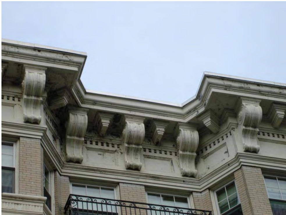
Detail at roof cornice
