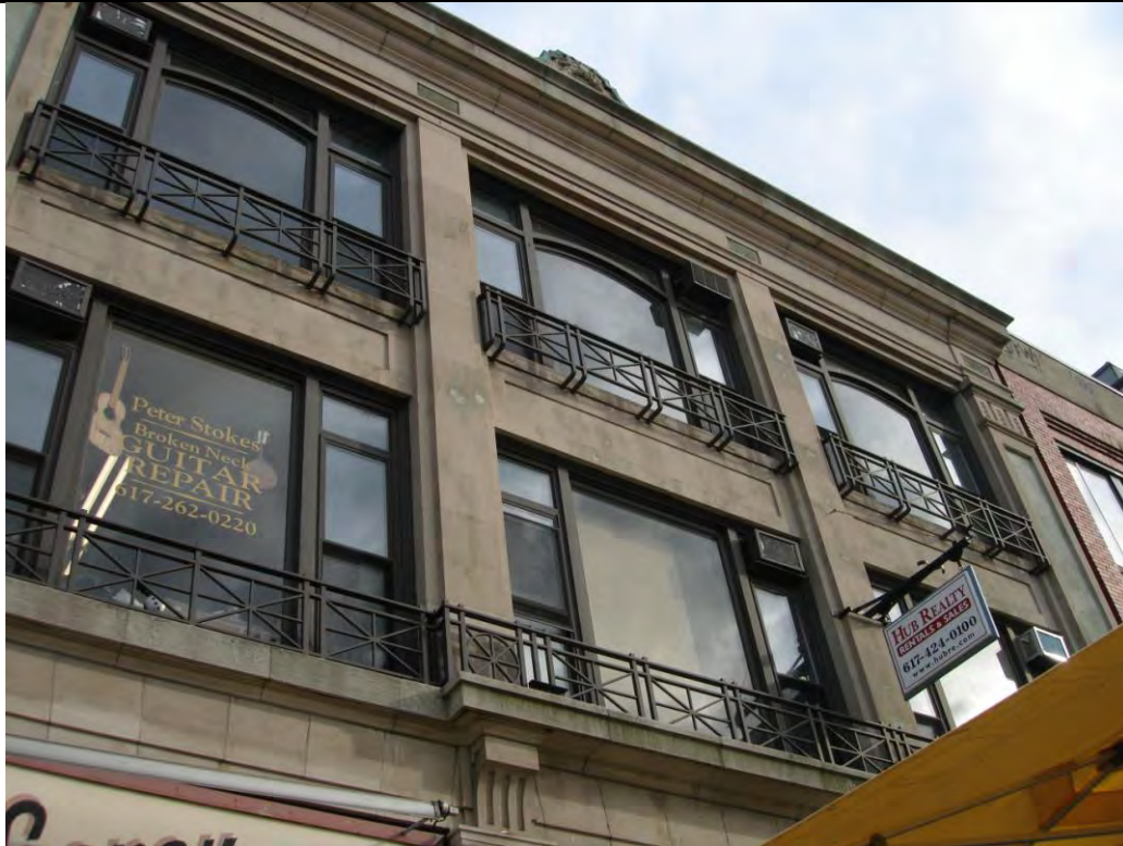
Front façade – second and third stories
