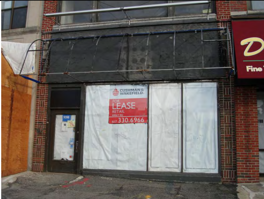
First floor --Notice original tapestry brick on sides and new brick veneer above first floor
