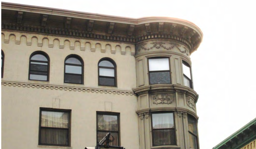
North-east corner detail
