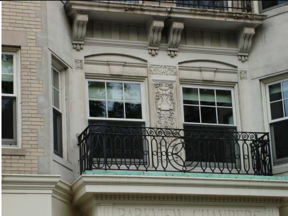
Detail at second floor balcony
