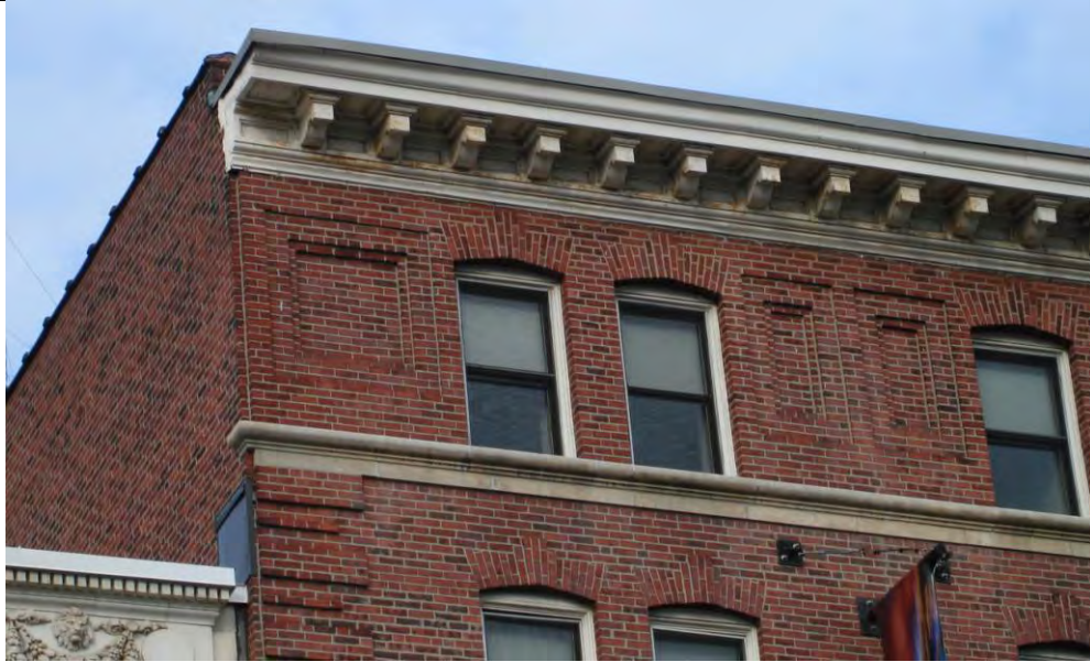
Detail of sixth floor and roof cornice
