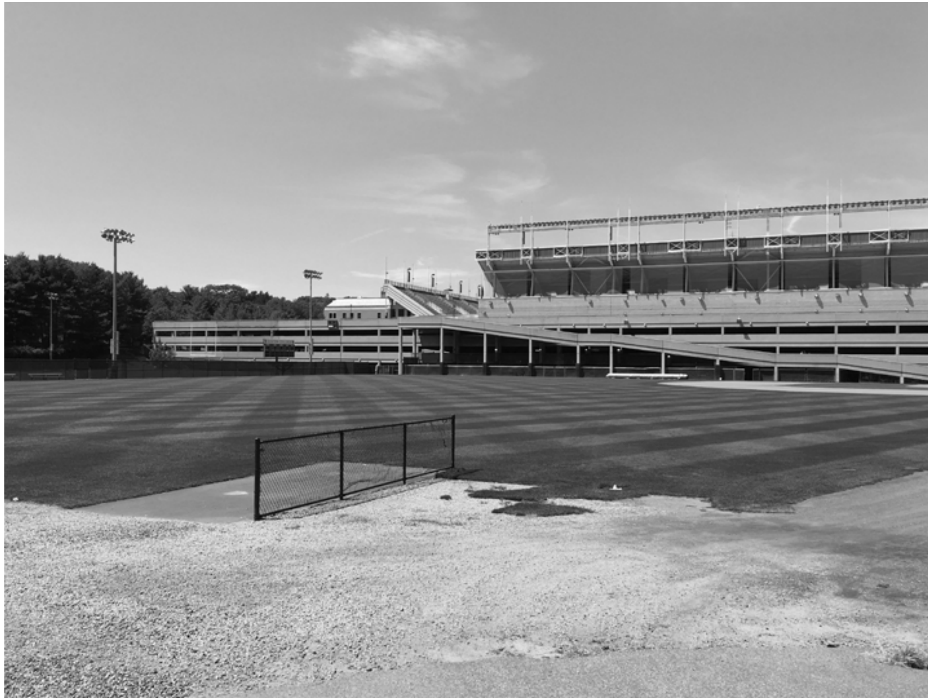
View of Beacon Street Parking Garage, Practice Field and Shea Field, east elevation from Pine Tree Preserve, facing SW
