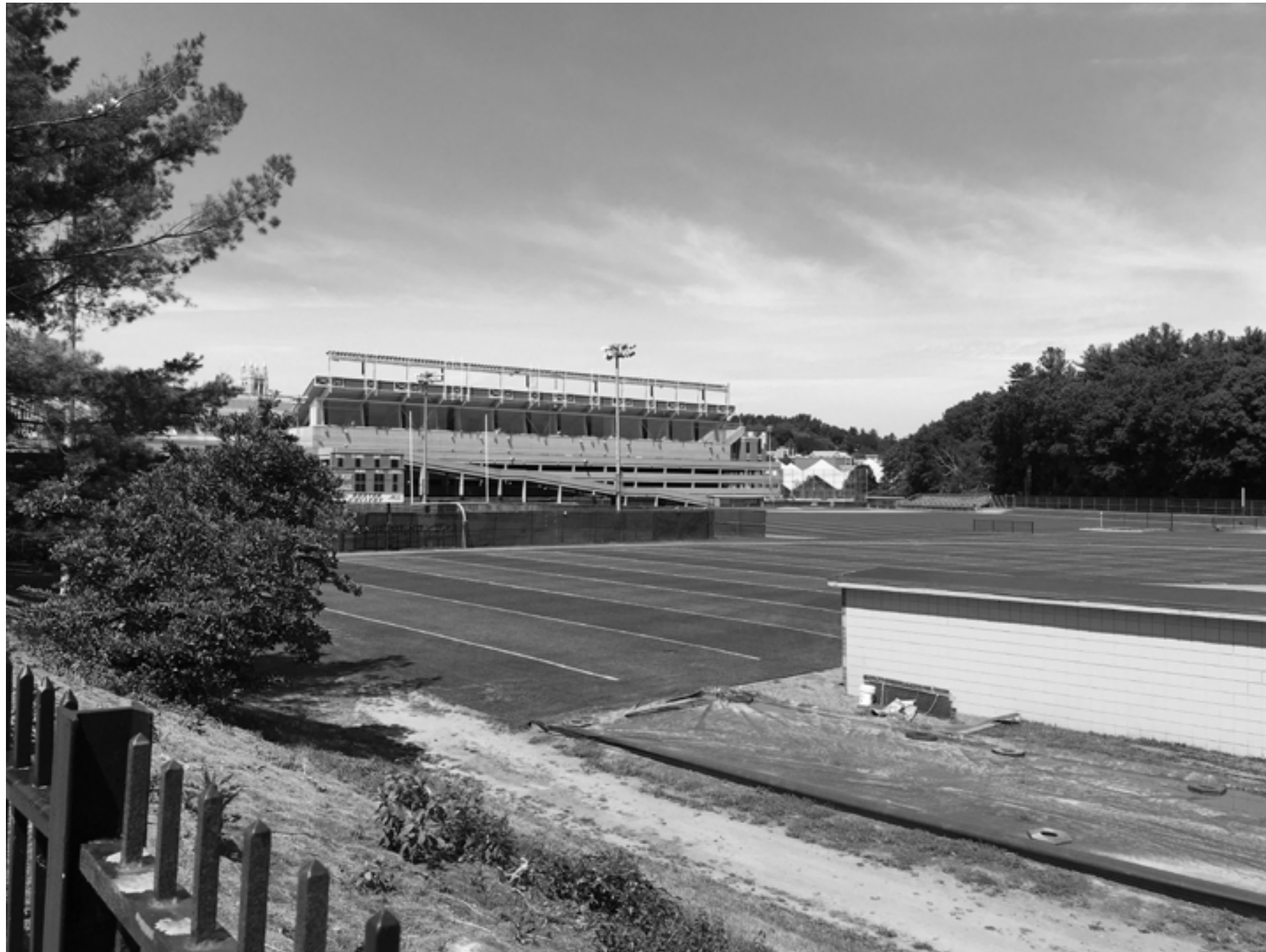
View of Beacon Street Parking Garage, Practice Field and Shea Field, east elevation from Beacon Street, facing NW
