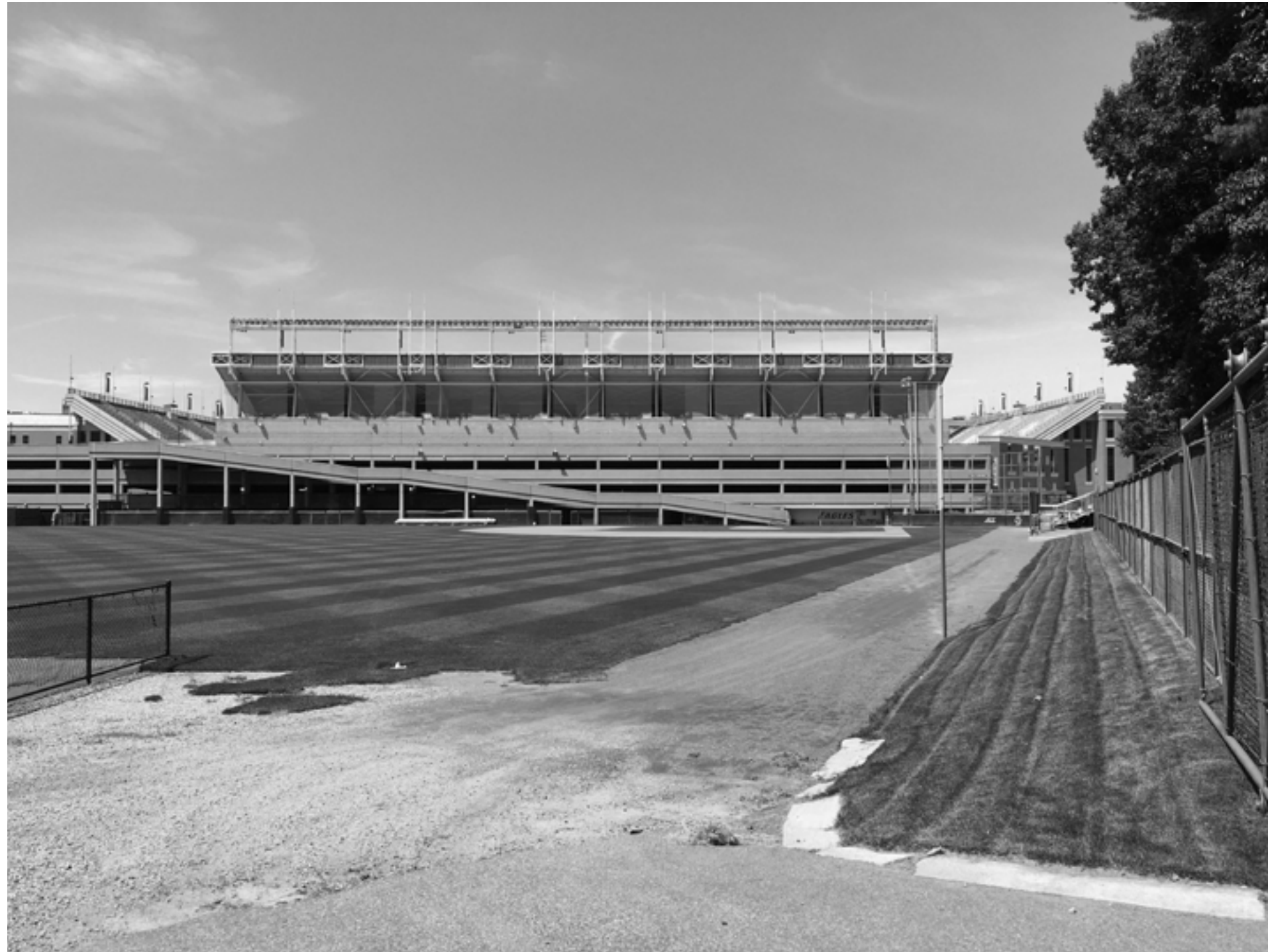
View of Beacon Street Garage and Shea Field, east elevation from Pine Tree Preserve, facing W
