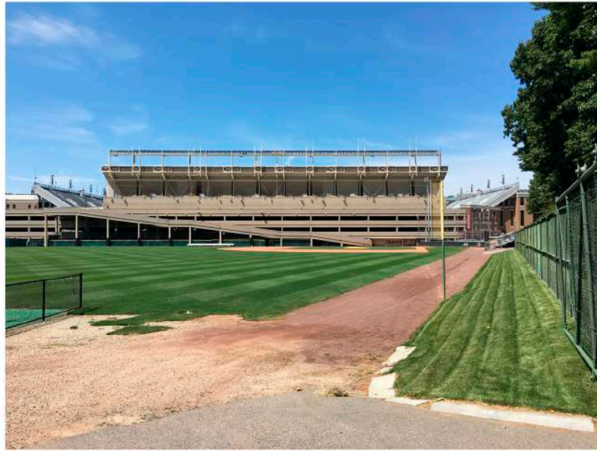
View of Beacon Street Garage and Shea Field, east elevation from Pine Tree Preserve, facing W
