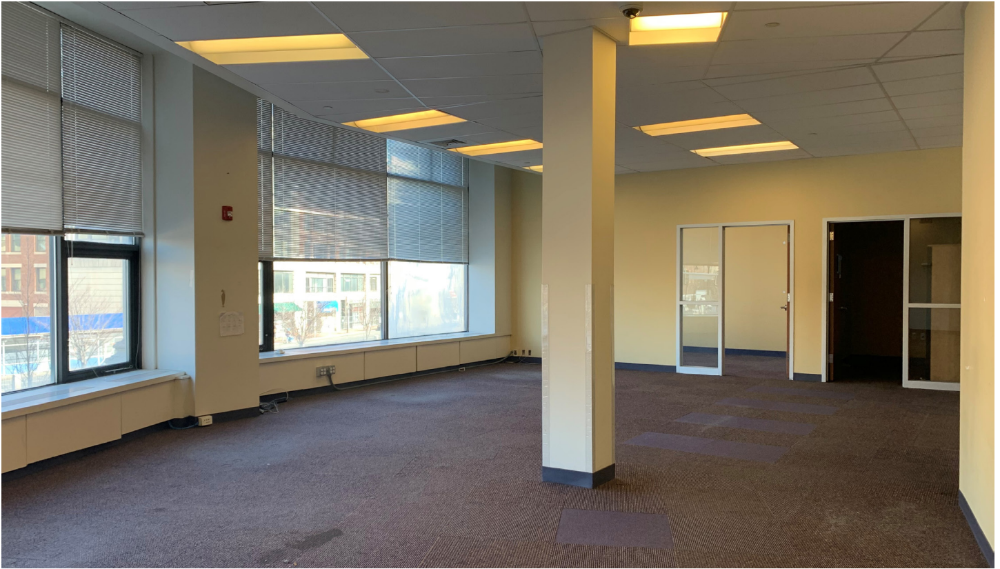
Interior View 1: North-facing instructional space
