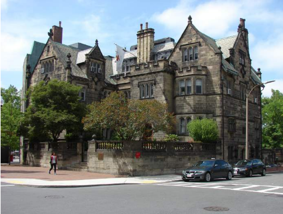
Photograph 1: View of front facade looking north
