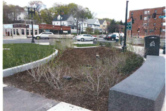
Rain gardens treat stormwater runoff from street and public plaza at Peabody Square in Dorchester
