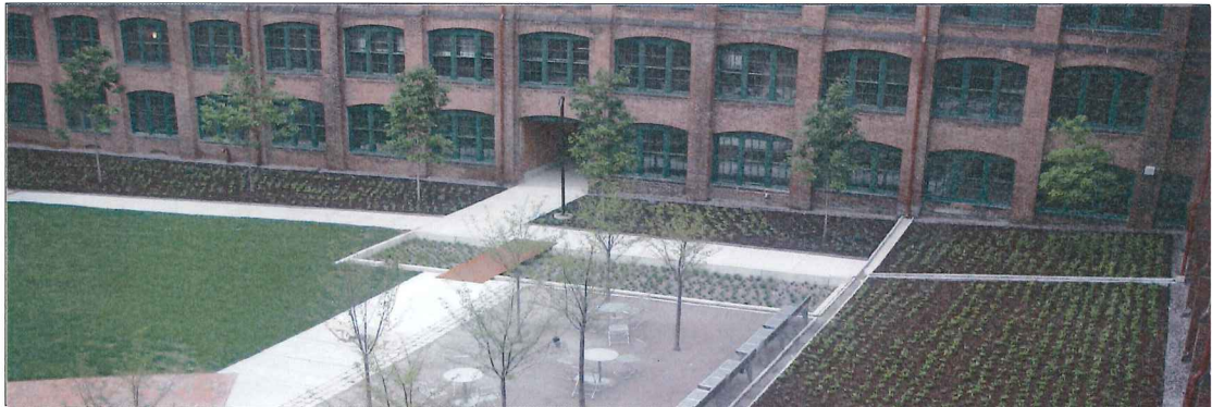
The Waltham Watch Factory Lofts in Waltham, MA. Designed with CRWA Blue Cities concepts, this mixed-use development filters stormwater before it drains into the adjacent Charles River.
