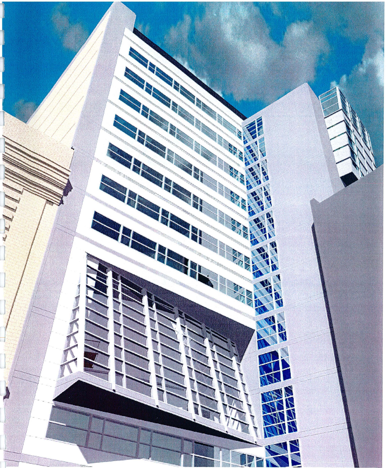
Tufts Performance & Production Center, 10 Boylston Place
