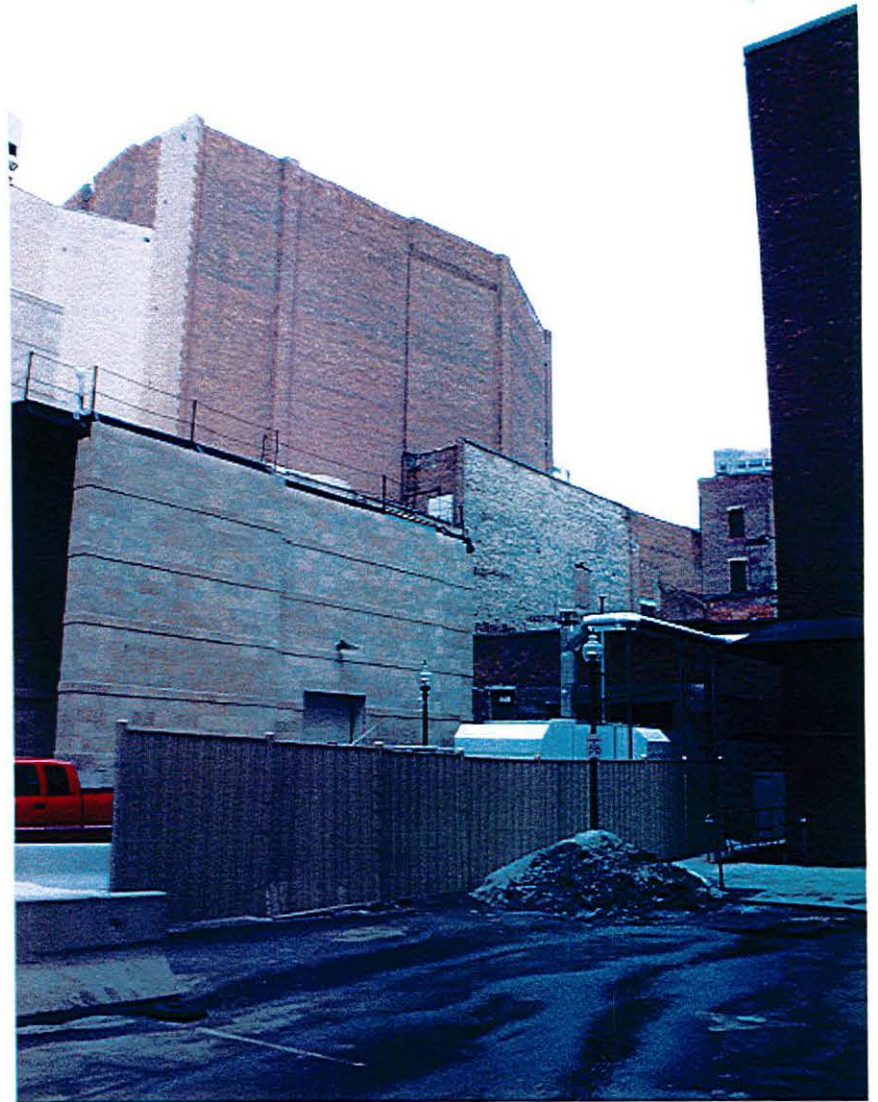
North Parcel at rear of Arcade Building
