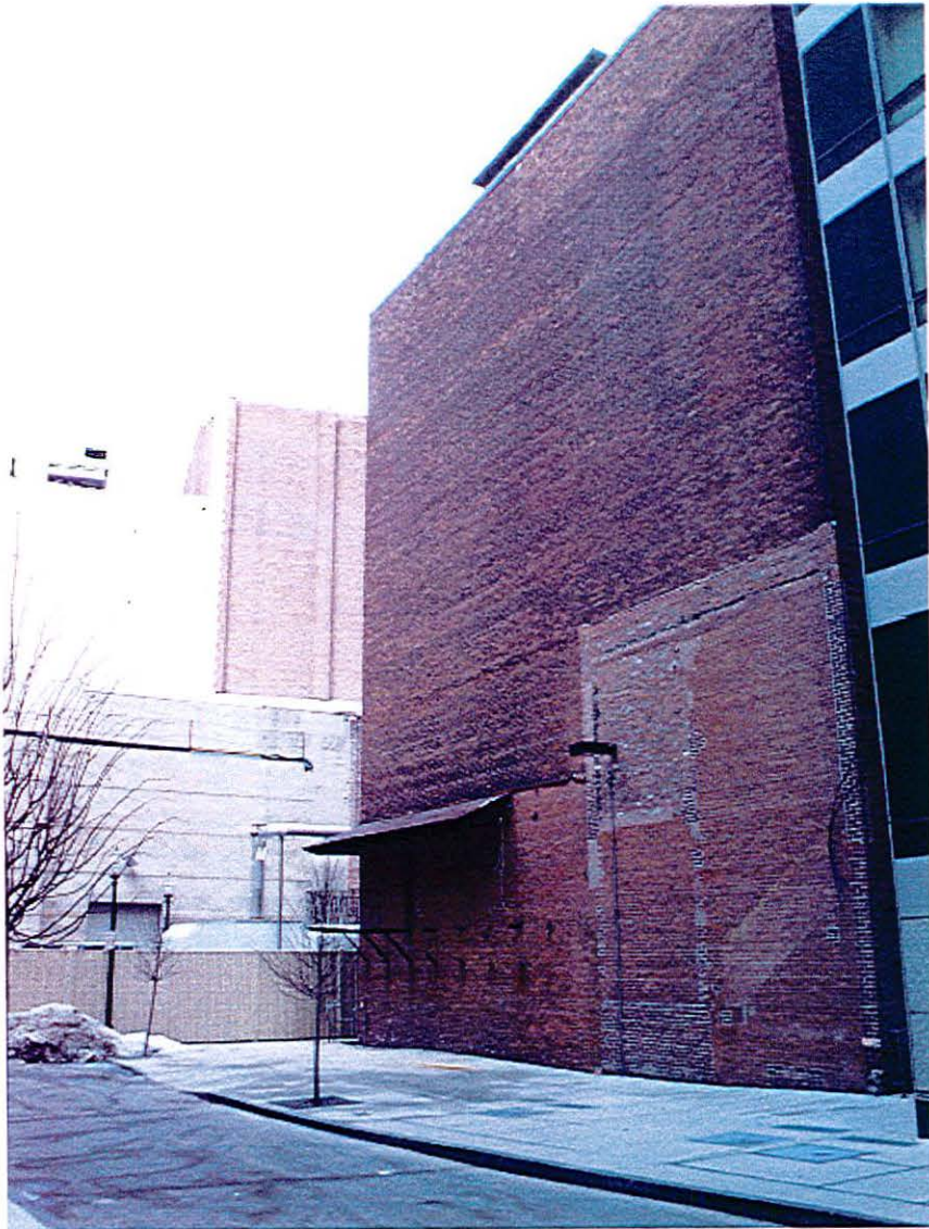
Rear wall of Paramount Theater
