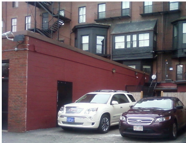
Red Cinder Block Wall Facing Rear of 116 Beacon
