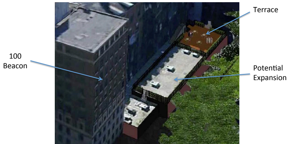
Fisher Mall Aerial Photo Showing Fencing around the entire Mall Roof
