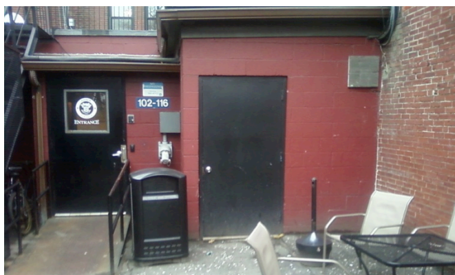
Red Cinder Block Wall at rear of 116 Beacon (Entry to the Mall)
