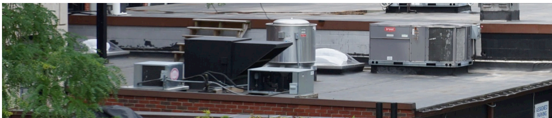
102 Beacon Roof Showing 7 roof additions
