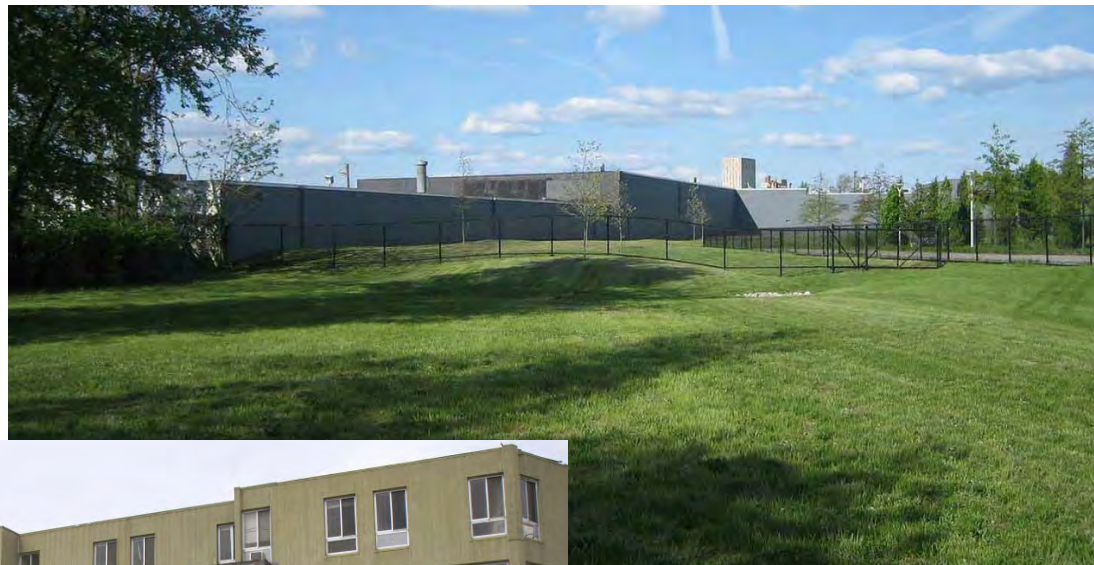
Construction of the Rena Park storm drain is underway in response to the collapse last year.
