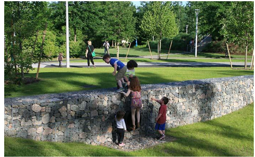
Drainage Wall & Bio-Infiltration Swale - Rena Park
