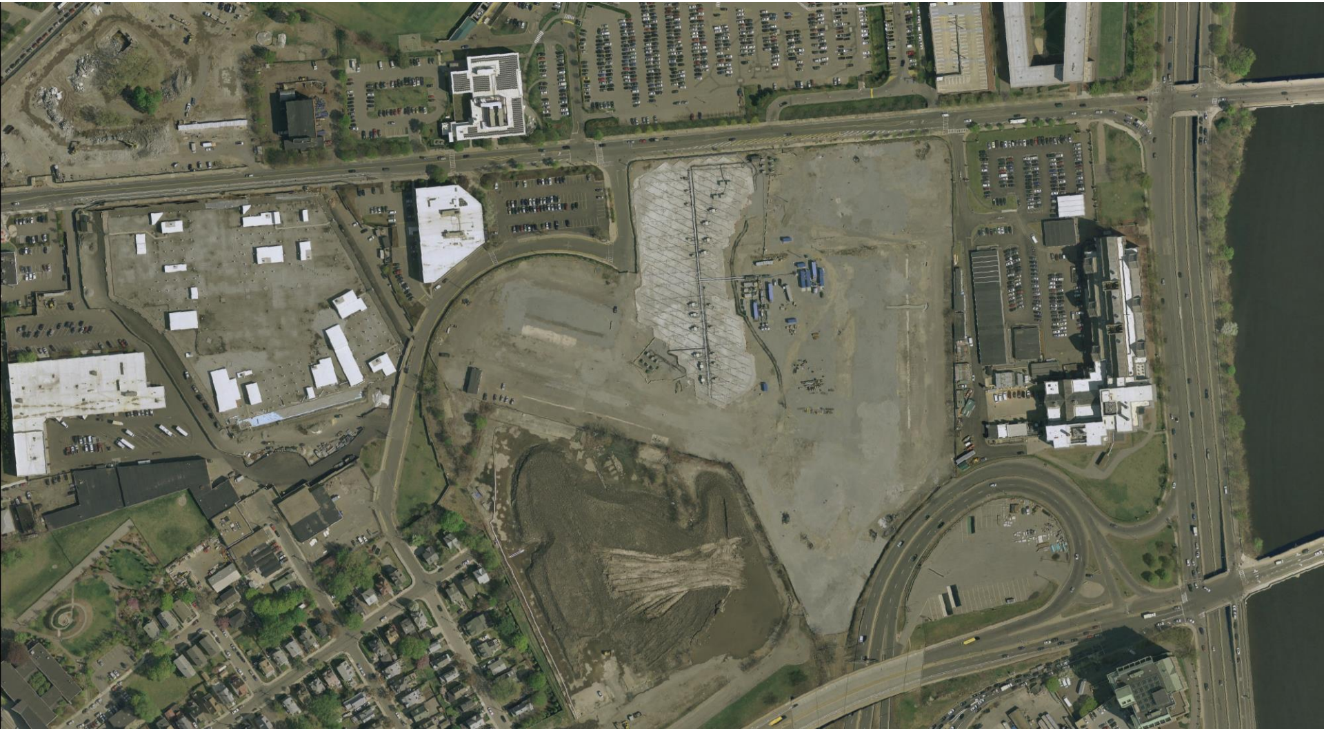
2015 Electric Resistance Heating
