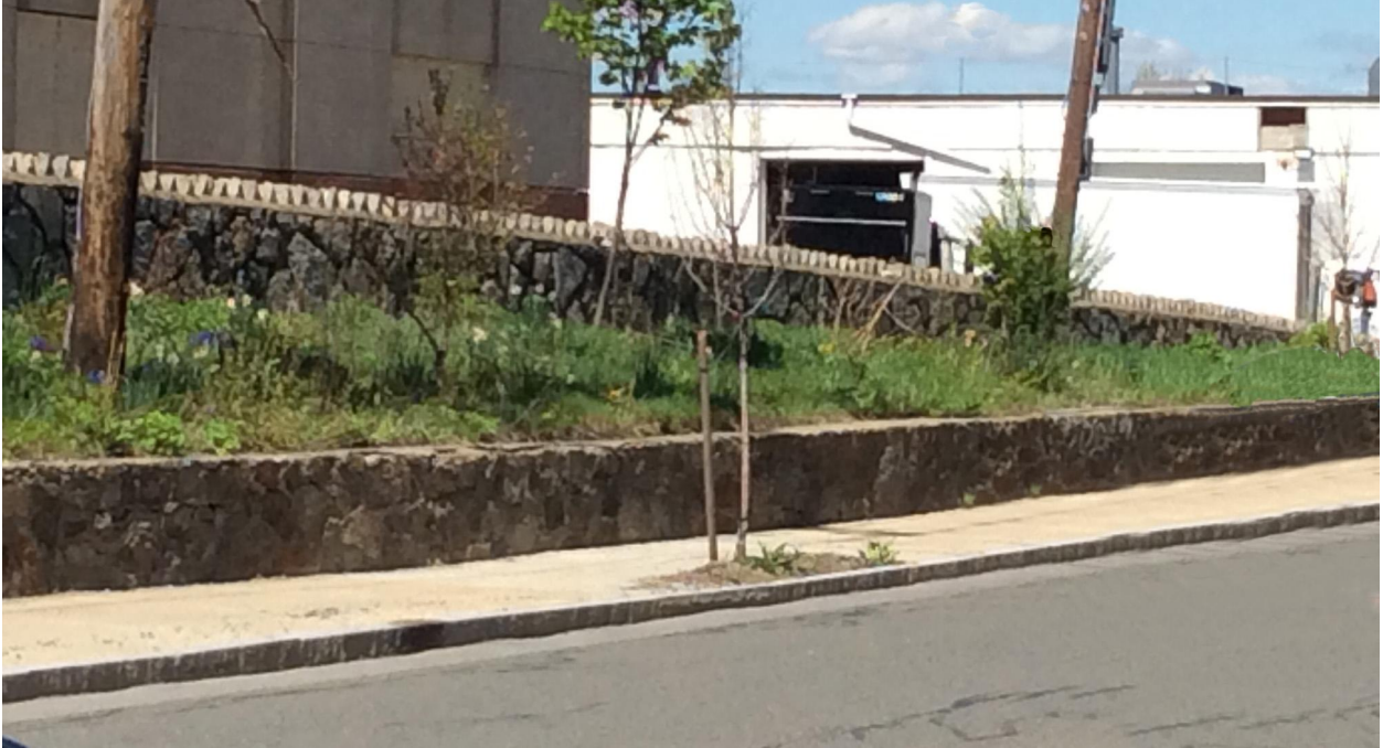
Everett St. Embankment looking NW
