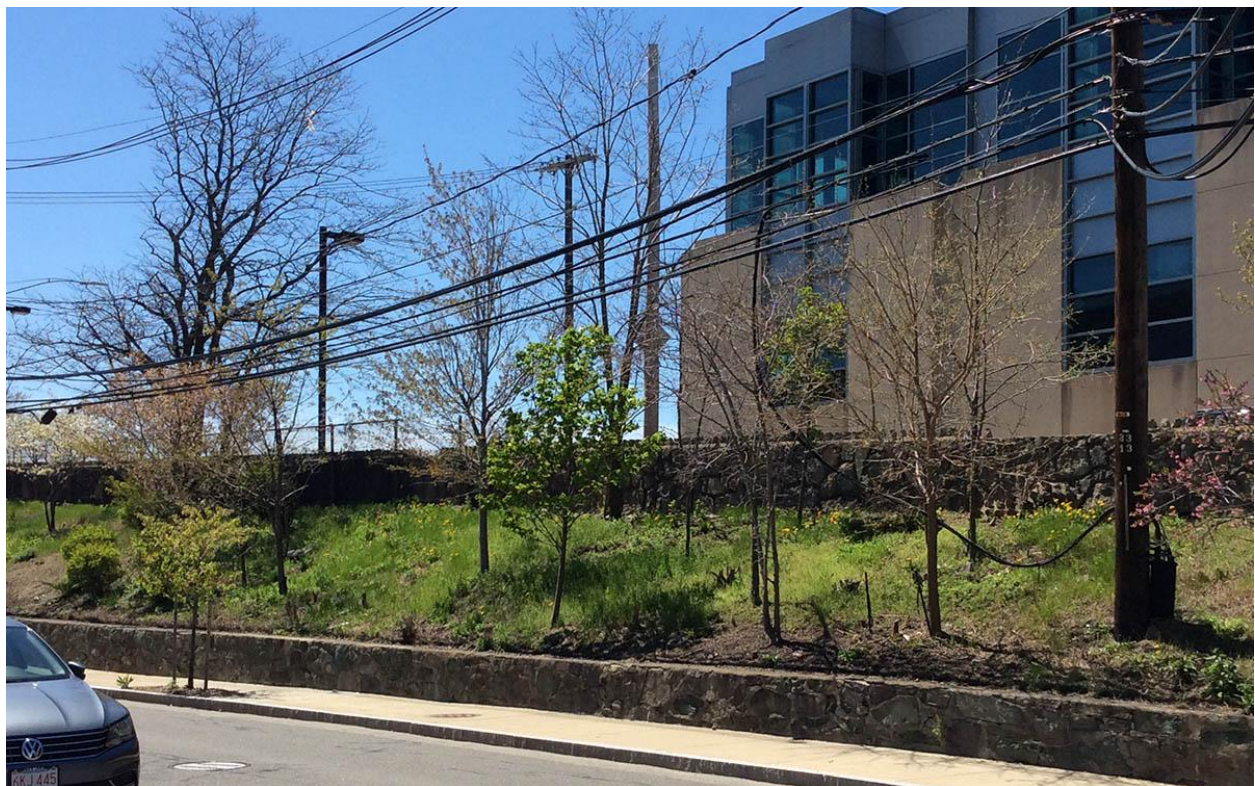
Everett St. Embankment looking SW
