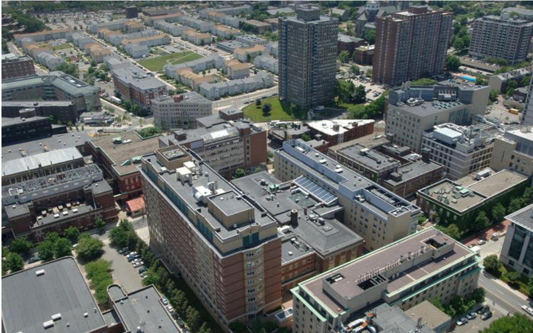
Center of Photo: Main Building Complex. Left to Right: The Fennell/Iorio Building, the White Building, and the Matricaria Building.
