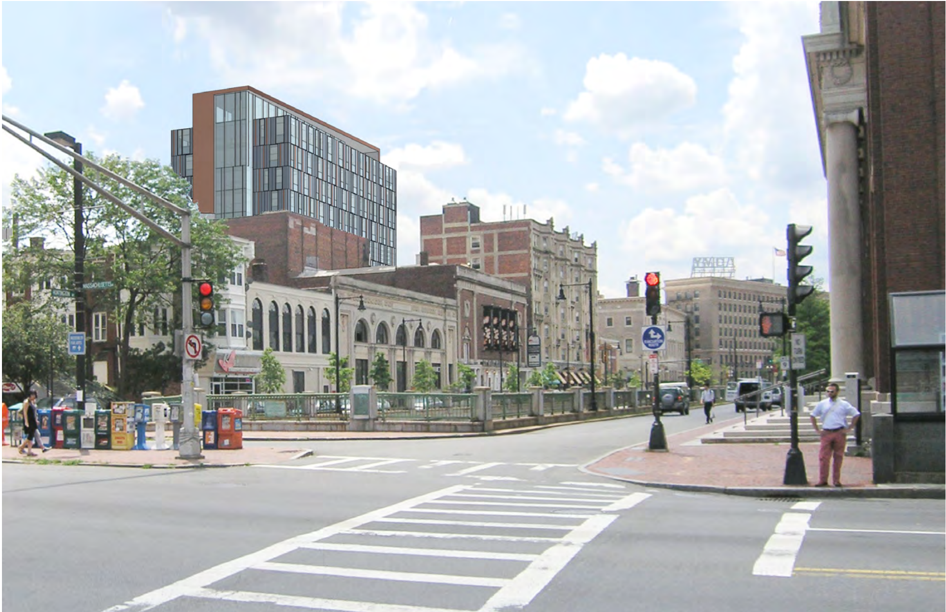
Figure 4-4 - View from Symphony Hall and Massachusetts Avenue Phase I - Student Life & Performance Center Project
