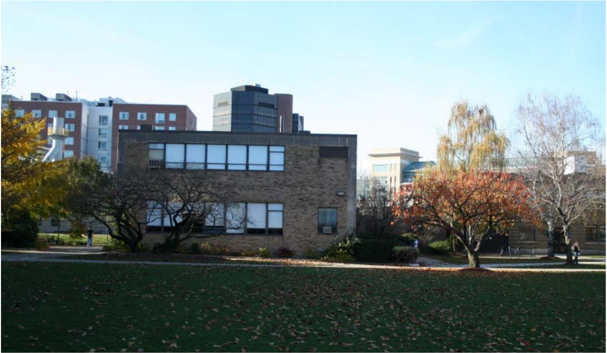
Figure 11: Willson and Kingman Halls (Buildings 7 & 6)
