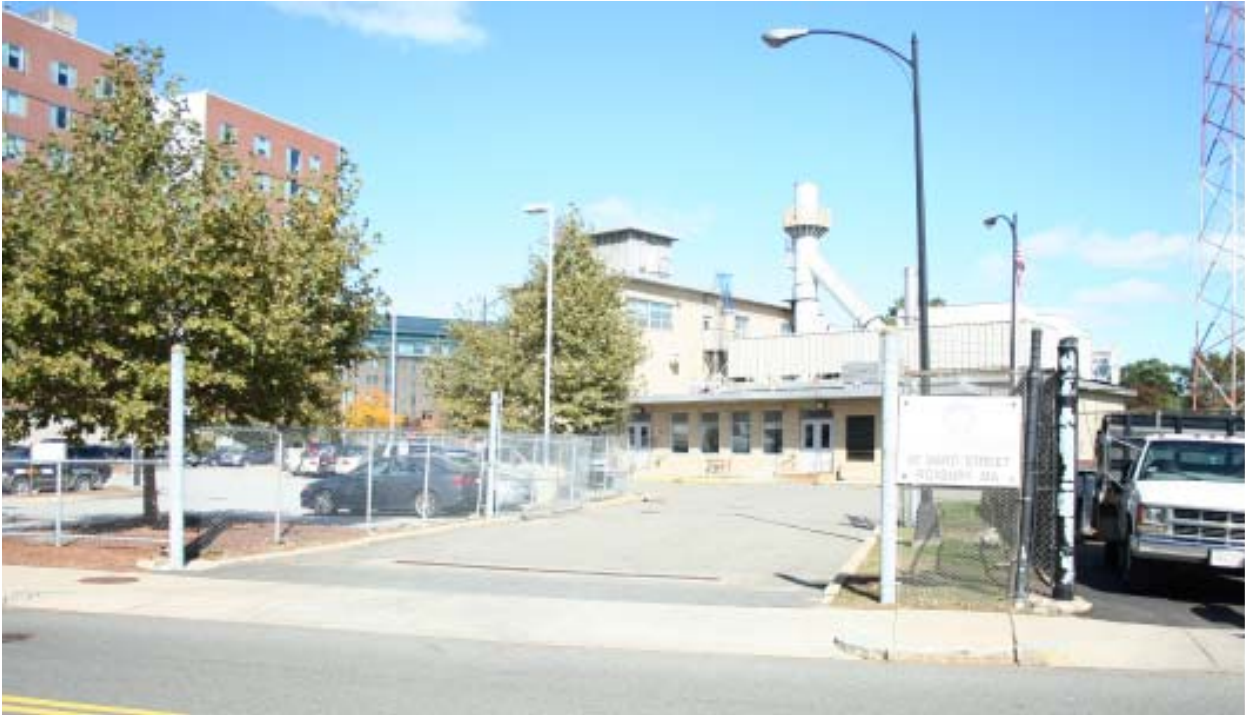
Figure 6: The Ward Street entrance of the Massachusetts Water Resource Authority Headworks
