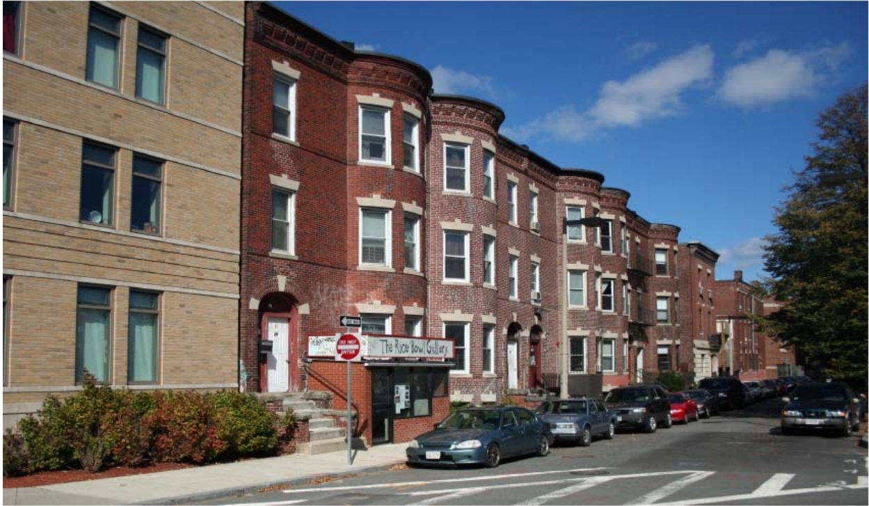
Figure 21: Vancouver Street properties adjacent to 555 Huntington Avenue
