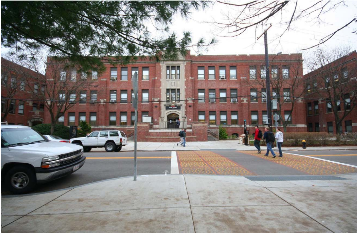
Figure 7: The Wentworth Annex located on the south side of Parker Street
