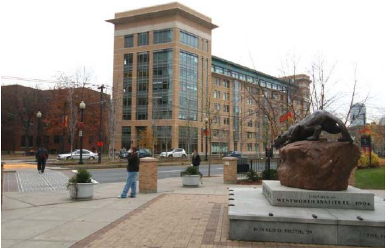
Figure 20: 555 Huntington Avenue, Building 12 viewed from Leopard Park
