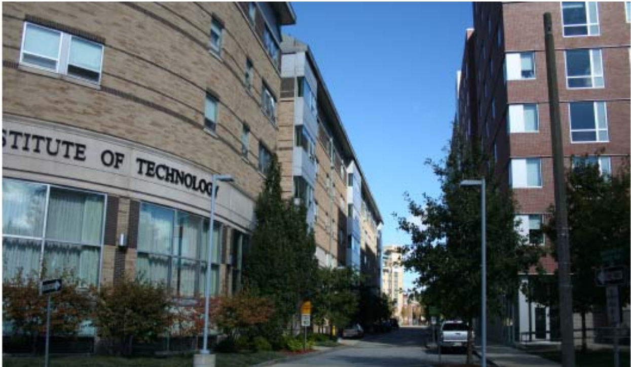
Figure 5: Wentworth's 610 Huntington Avenue Residence Hall adjacent to the MassArt Residence Hall on the corner of Ward and Vancouver Streets
