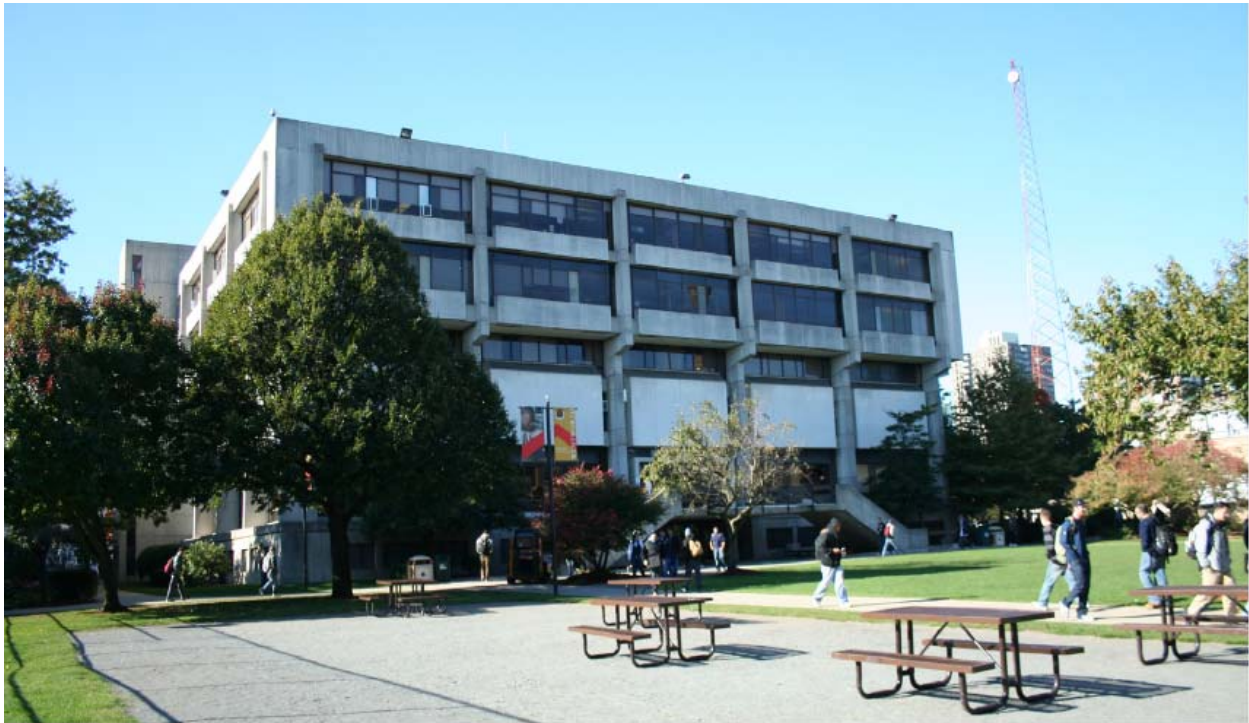
Figure 12 Beatty Hall, Building 8
