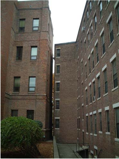
Photo taken by Sarah Nailor Exterior wall of buildings 122 Riverway Square Condominiums and Wheelock Library / Rear View as taken from 25 Pilgrim Road- Wheelock surface lot
