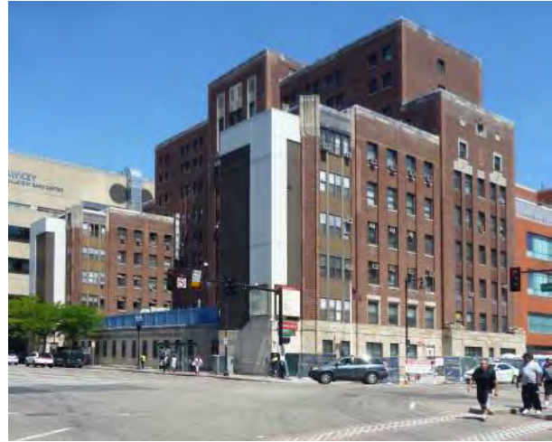
2. Massachusetts Avenue and Albany Street looking North.
