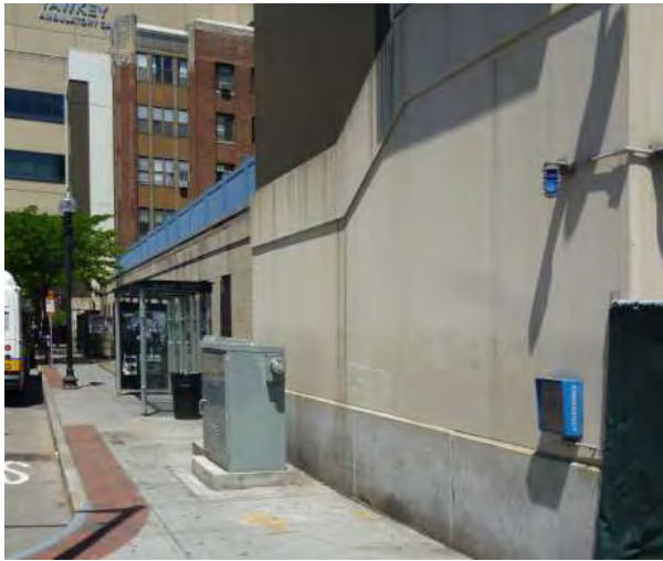
1. At grade along Massachusetts Avenue looking North.
