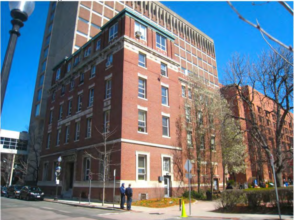
b.1 A Building
