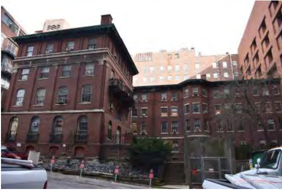
1. Southwest elevation of Vose Hall
