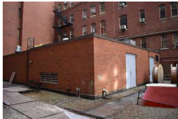
4. One-story Betatron attached to the northeast elevation of Vose Hall.
