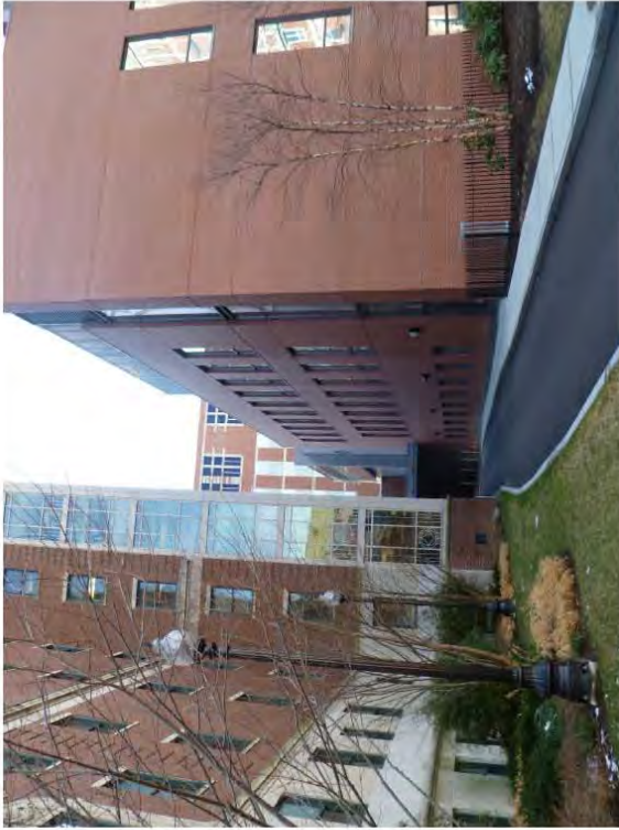
Photo 4: View from East Concord St. looking southwest. Shapiro Drive exit with East facade of Moakley Cancer Center on right and 85 E. Concord on the left.
