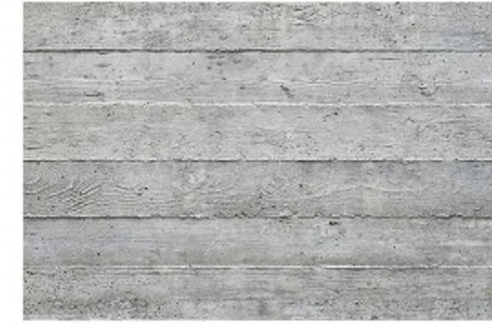
BOARD-FORMED CONCRETE FOUNDATION
