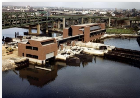
Figure 4-10. New Charles River Dam (NCRD).
