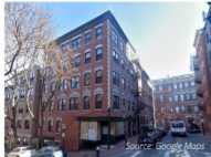
15 Revere St, Beacon Hill - 10 Units
