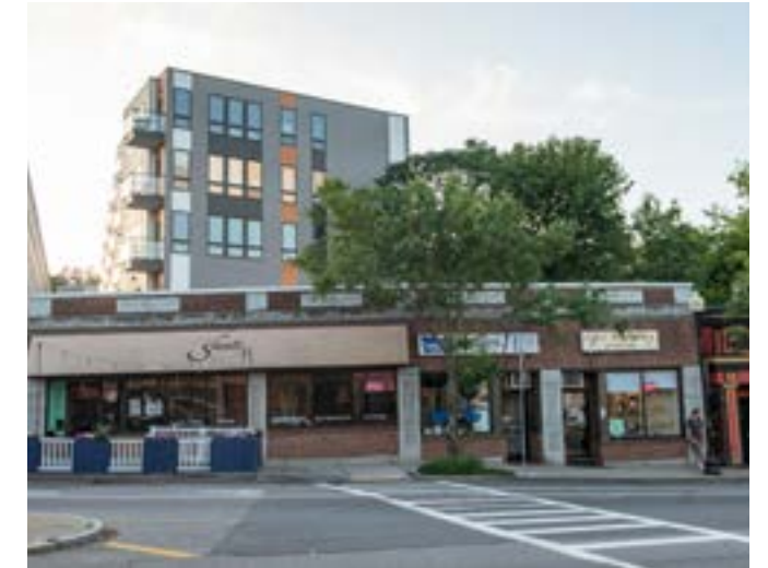
Residential and Commercial along Washington St
