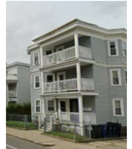
Example of a flat roof
