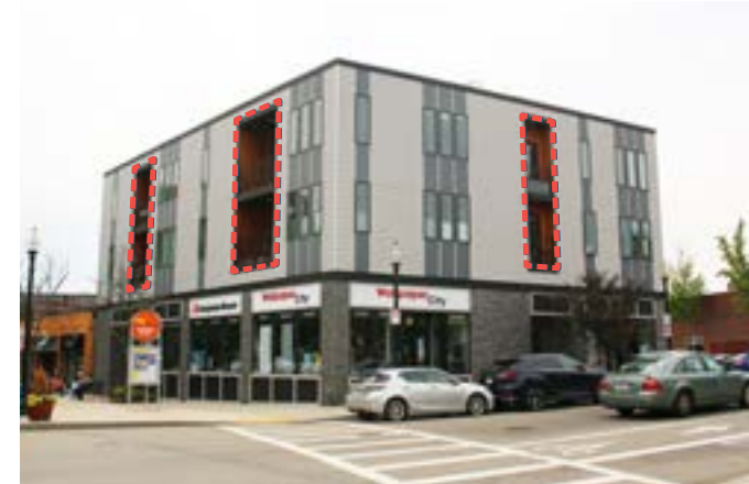
Recessed balconies for residential units above Wallpaper City
