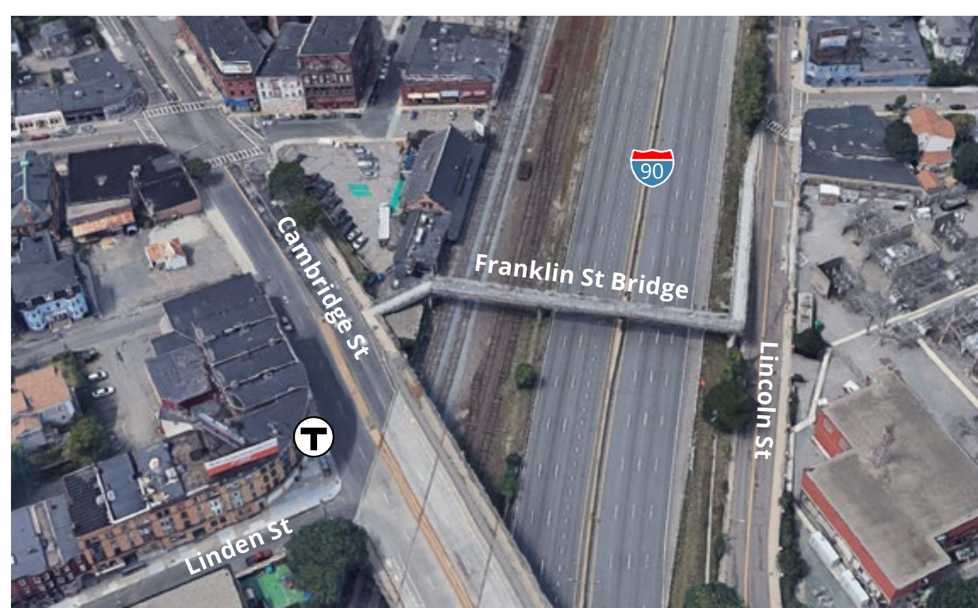
Franklin St Bridge - View from Cambridge St
