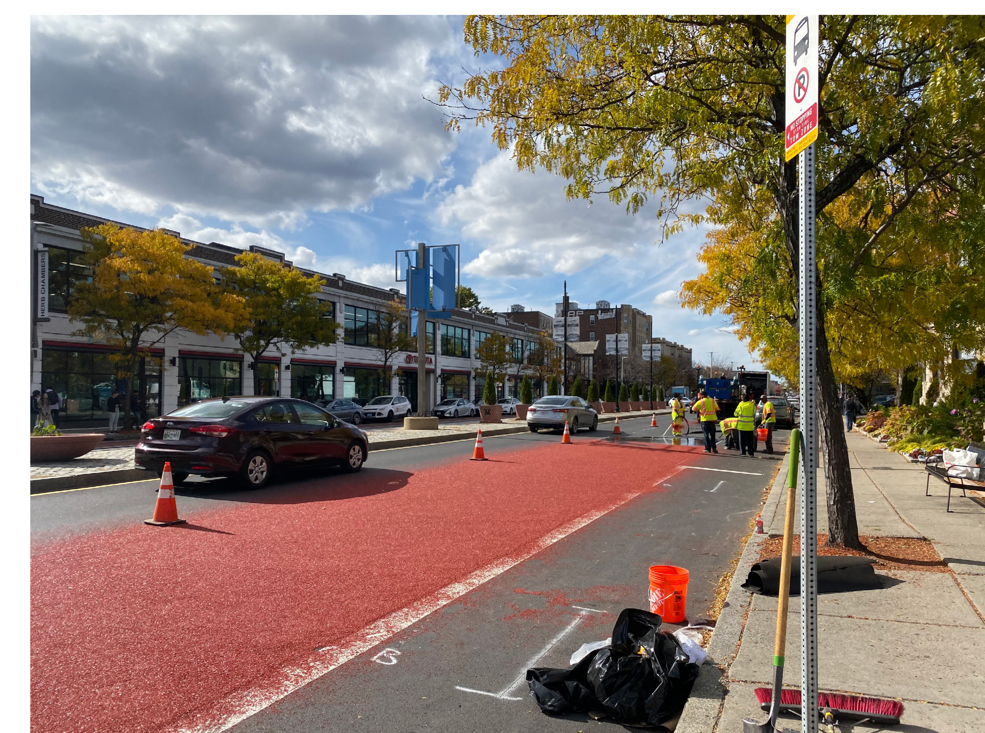
Image: Installation of the Westbound Brighton Ave bus lane.
