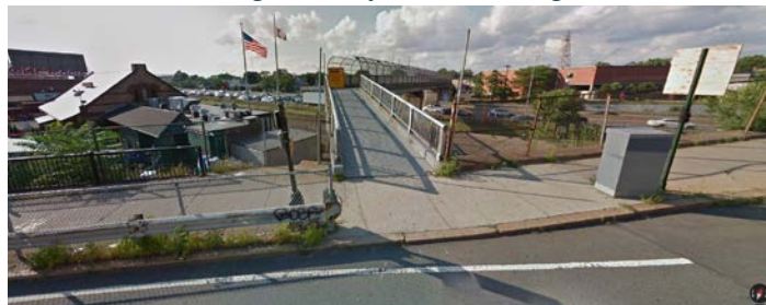
Franklin Street Bridge - View from Cambridge Street
