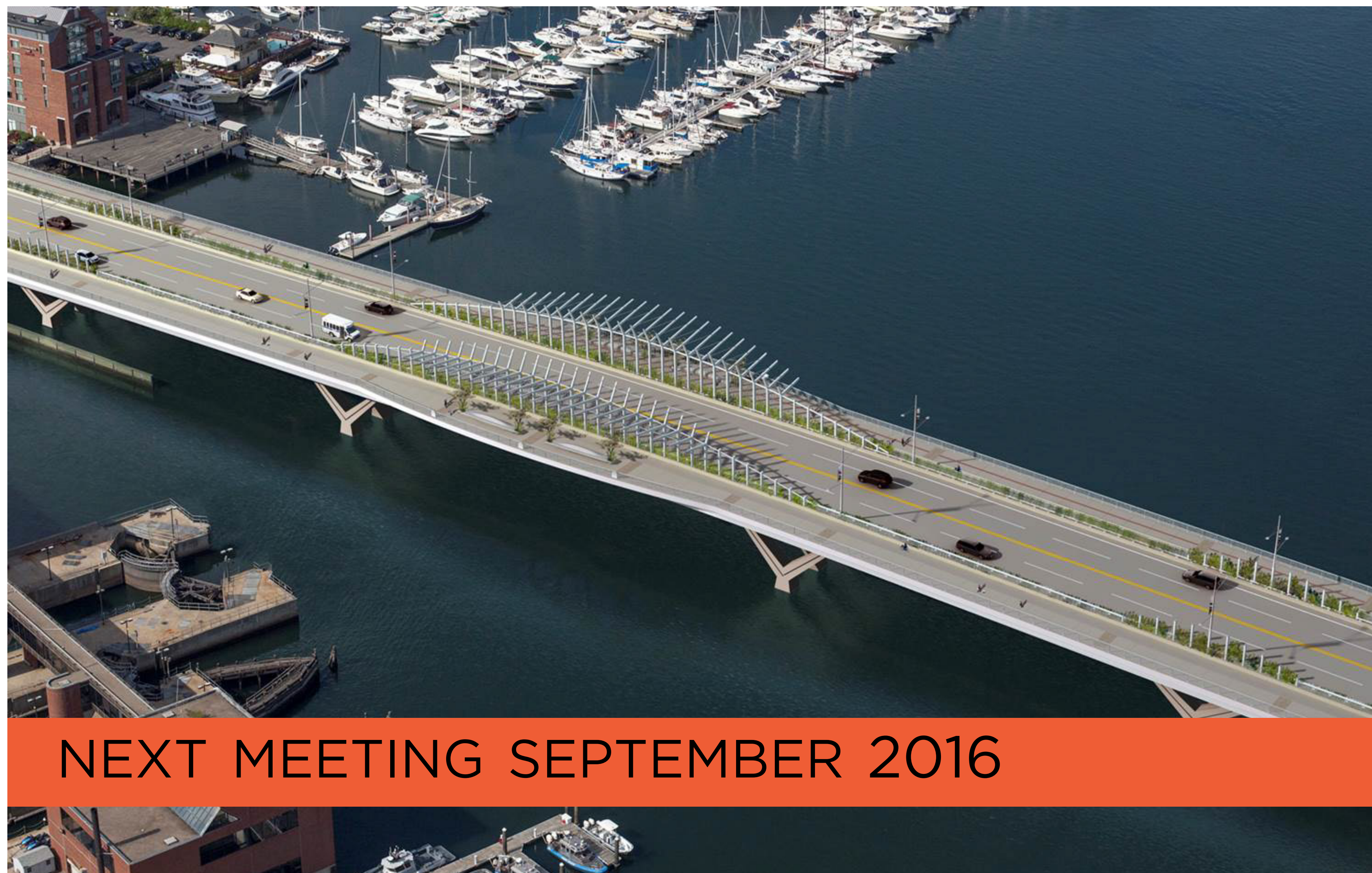
NORTH WASHINGTON BRIDGE
