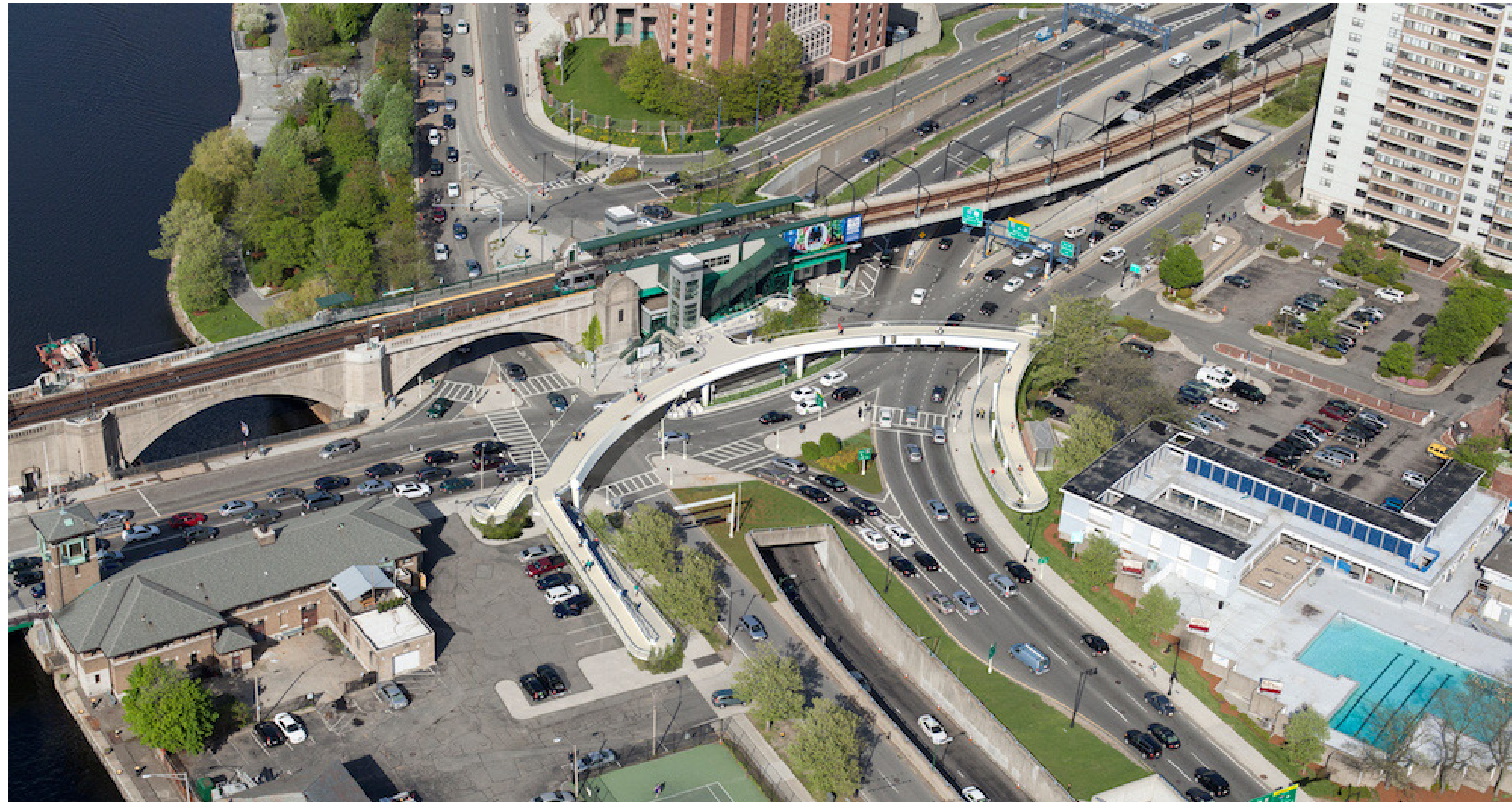
LEVERETT CIRCLE BRIDGE
