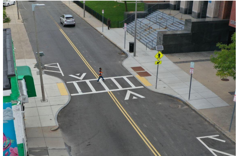
A raised crosswalk in Roxbury.
