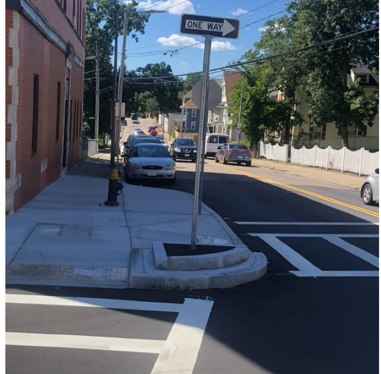
Curb extension in Dorchester.
