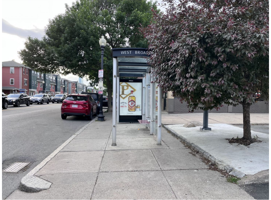
Bus Shelter at D Street and West Broadway
