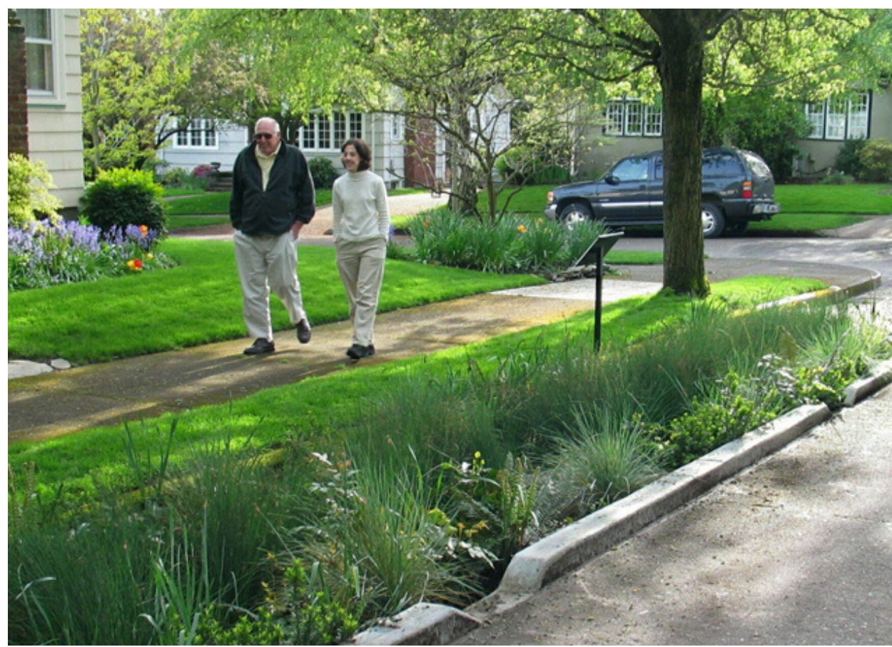
Slotted curbs source: American Society of Landscape Architects Bordillo con ranura Fuente: American Society of Landscape Architects
