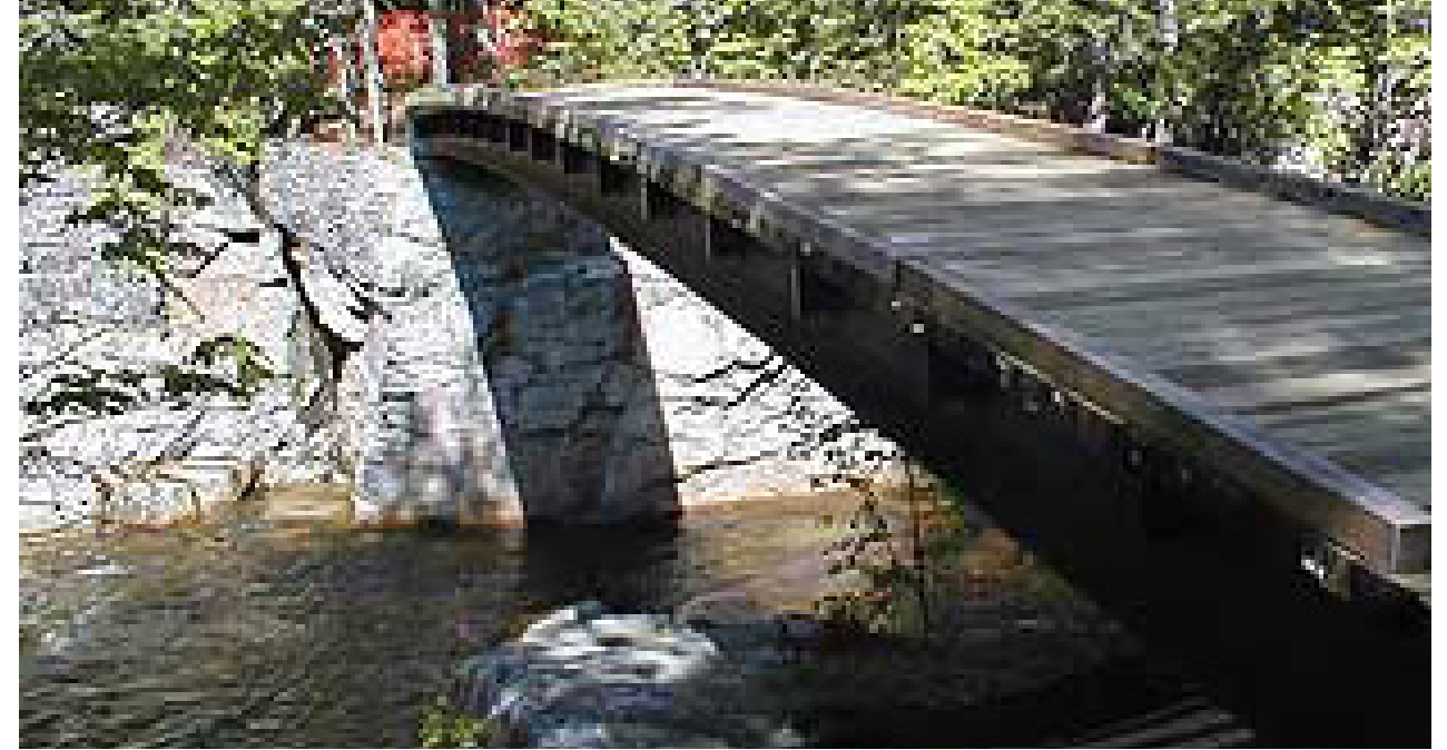
bridge over tidal well
