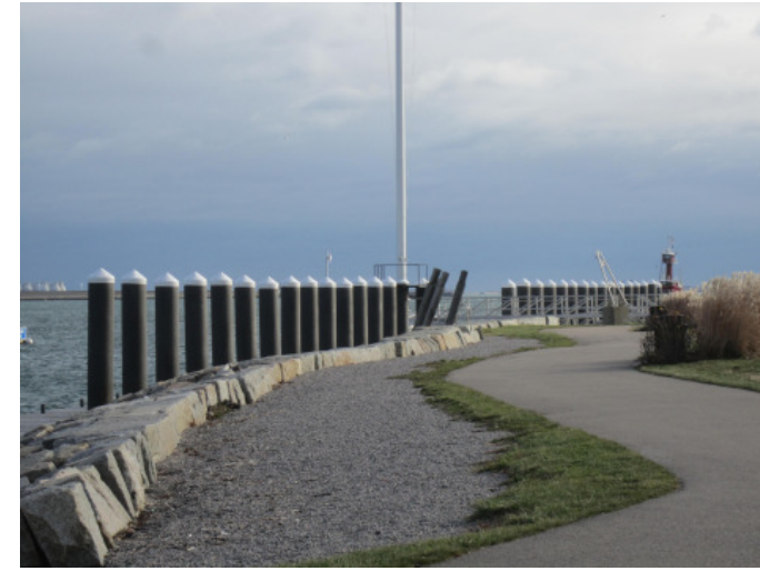
filtered view to the west
