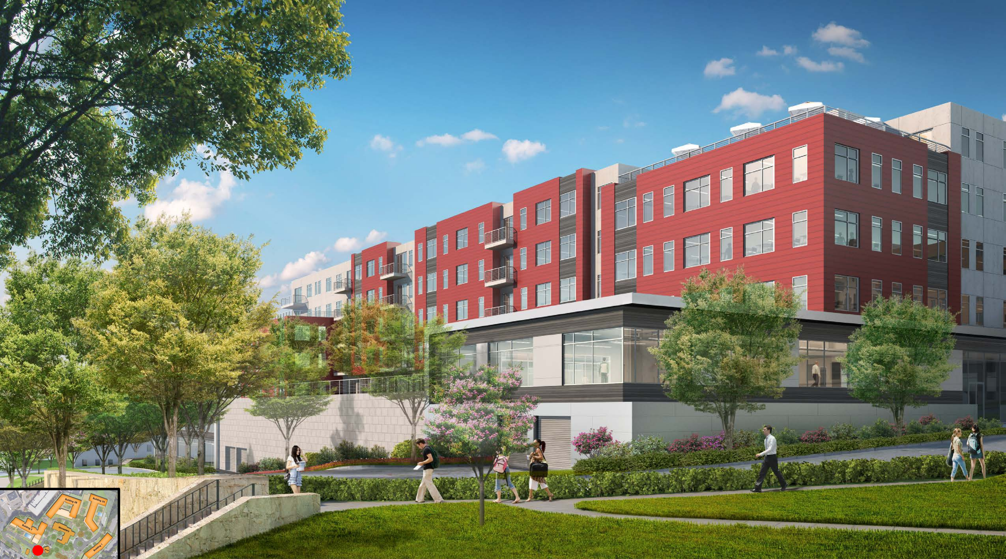
Front of Building 3
