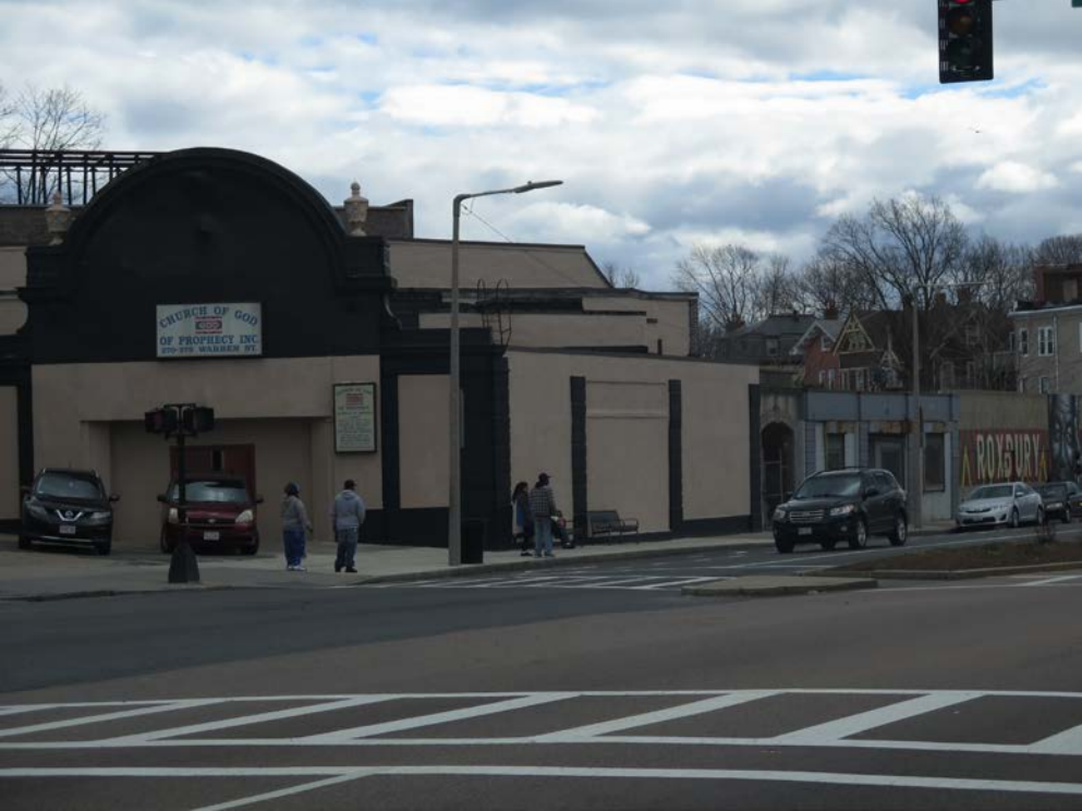
Adjacent to 270-272 Warren St. DND Owned Buildings along Warren St.
