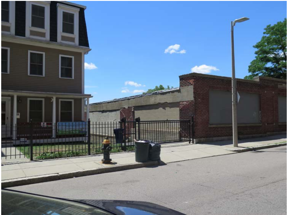
Adjacent residential building to vacant site bldg. along Waverly
