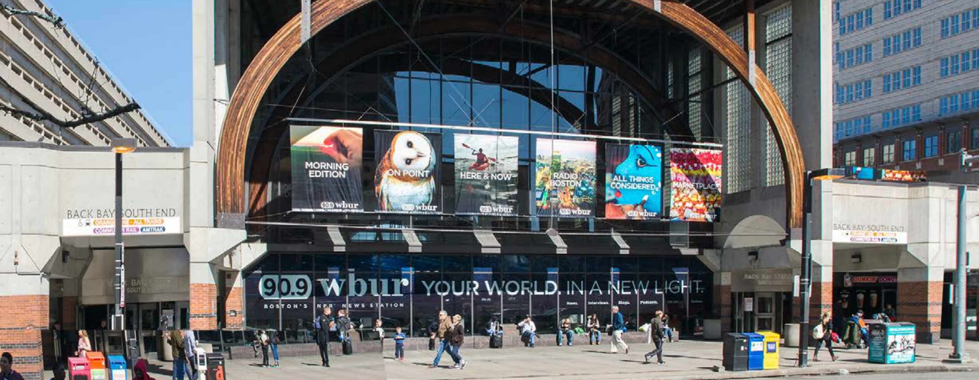
EXISTING STATION ENTRY (WEST)
