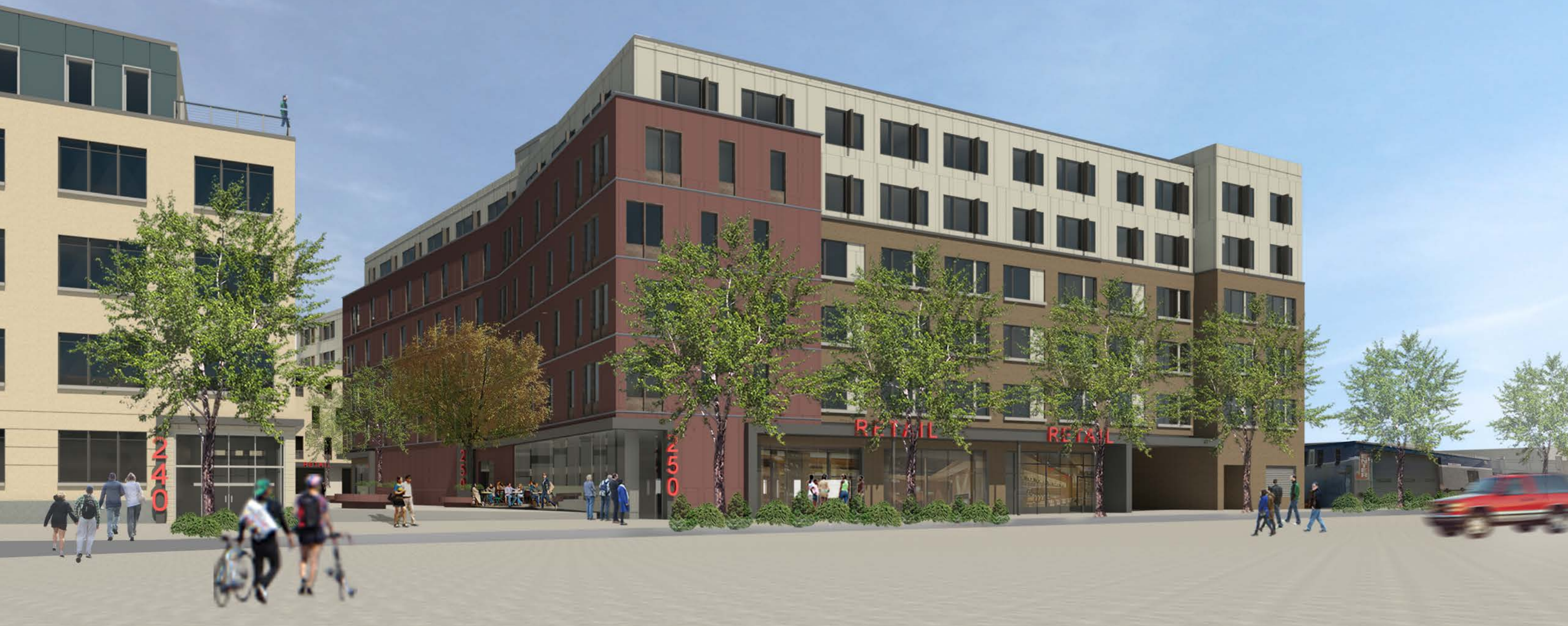
HANCOCK STREET - VIEW NORTH INTO SITE BETWEEN 240 & 250 HANCOCK STREET
